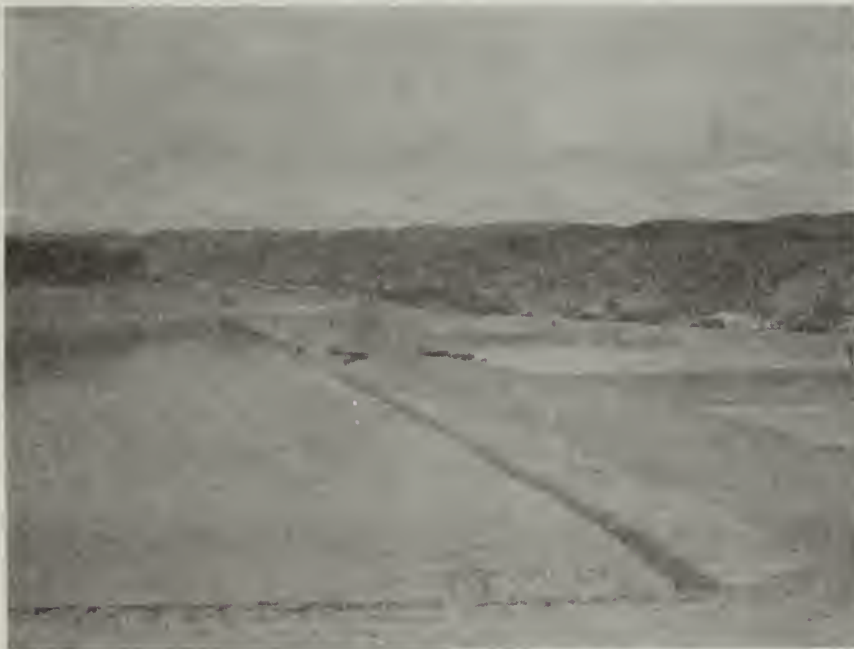
Figure 3-1-12. Phase III Ponds Complete
