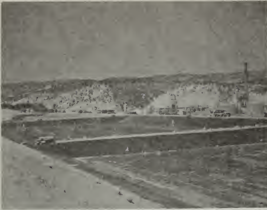
Figure 3-1-11. Phase III Pond Liner Installation
