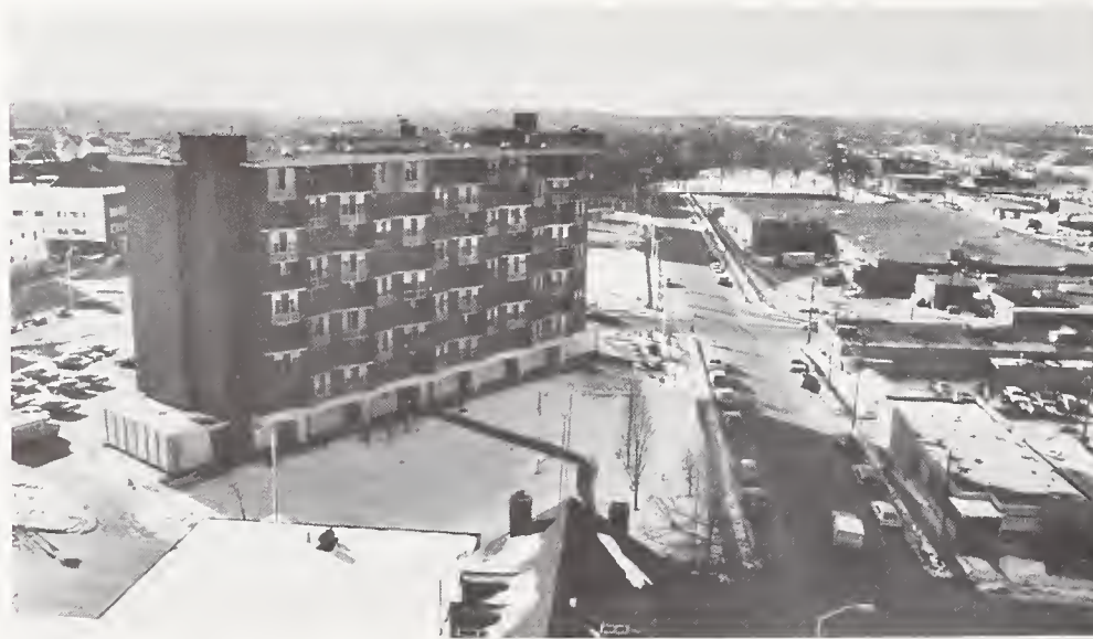
Residential Building (NBS)
