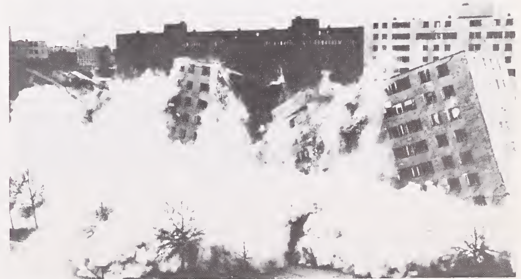
Pruitt Igoe—After (HUD)
