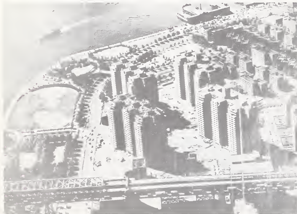
Community Separated from Surrounding Area (HUD)
