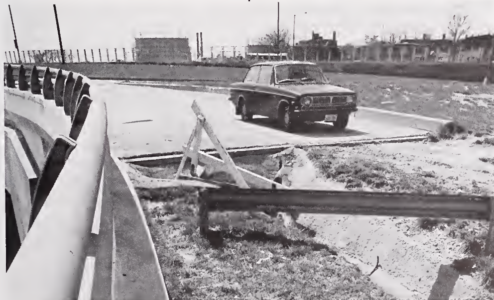
Uncompleted Highway (NBS)
