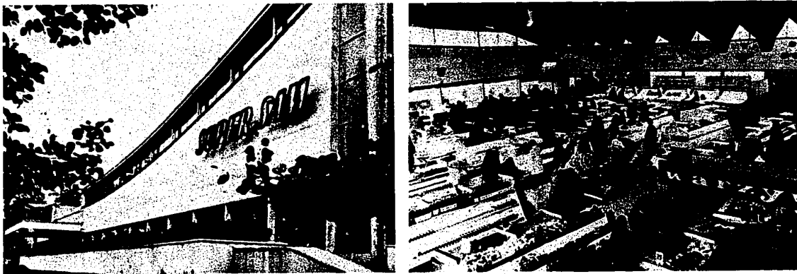
FIGURE 29. Supermarket in Warsaw (U/OU)
