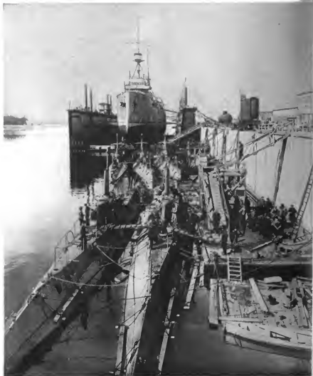
The photograph reproduced above shows part of the Canadian shipyard at Maisonneuve, near Montreal. A British man-of-war is in the floating drydock and in the foreground are five of the submarines constructed there, preparing to go to sea. Five others, completed early in the summer, have already proceeded to the Dardanelles and aided in the Allied attack.
