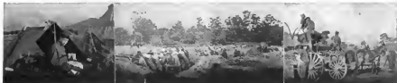
Student in shelter tent camp; instruction is given in digging trenches; the knack of loading wagons is taught by practice
