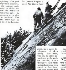
Swiss army engineers building road in the Alps
