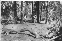
Reconnaissance showing Biltmore stick in use. Crew engaged at logging, calipers, and recording diameter measurements.
