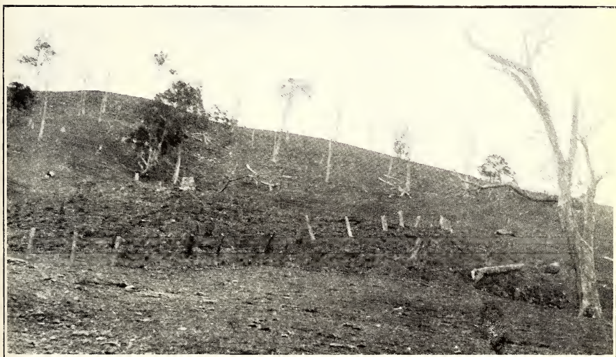
Fig. 2.—Landslide, which occurred in 1922, on southern slope of ridge eastward of Vault Hill, Picton.
