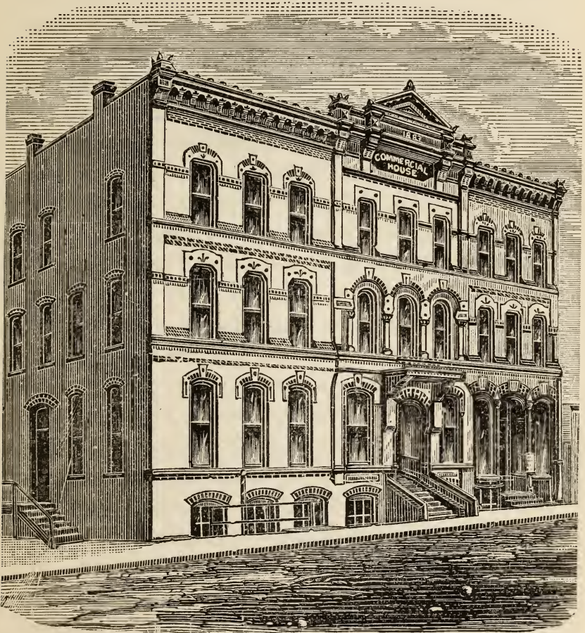
COMMERCIAL HOUSE, SIOUX FALLS.
