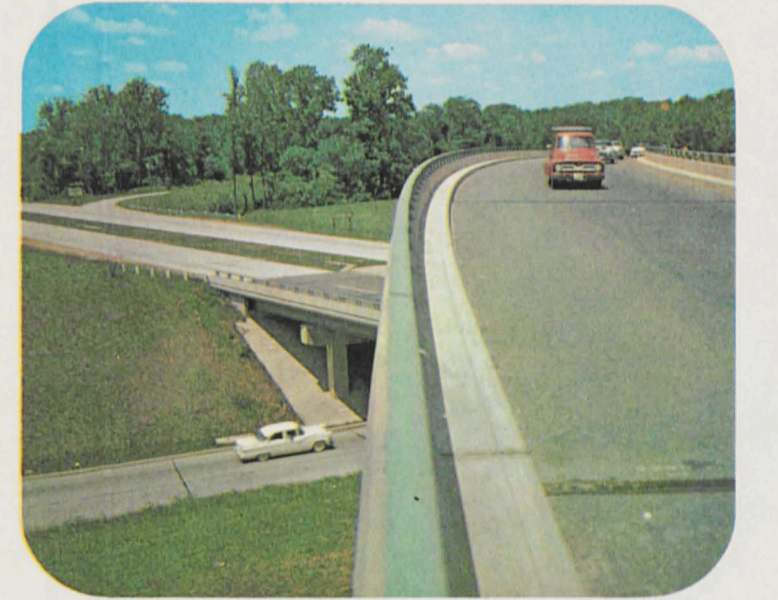
Tri-level traffic interchange—typical of the safety standards of Maryland highways.
