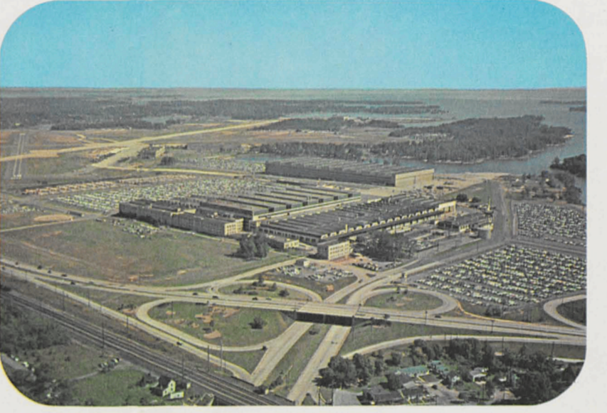
Modern Highways serve this Industrial Plant.
