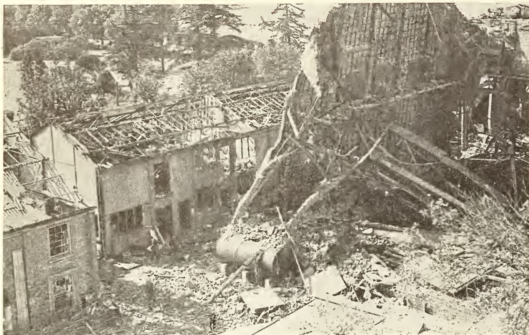
THE END of Warners' Teddington studio, England—temporarily. The scene above is of the devastation wrought by the robot bomb which hit a fuel oil tank and caused fire as well as blast, completely wrecking the plant and killing A. M. ("Doc") Salomon, British production chief, and two companions. Two others were injured.
