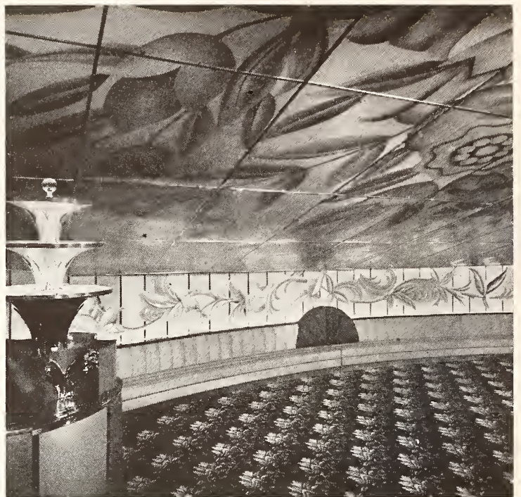
The main lounge is an oval room entered down a few steps. The built-in seat opposite the steps is 38 feet long. The wall and ceiling are made up of aluminum panels, which are attached by snap-on mouldings and ornamented with attached aluminum figures. Lighting is provided by a neon cove behind the seat.
