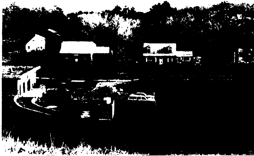
PHOTO NO. 13 - View of the immediate downstream area showing the Water Treatment Plant and the Maple Meadow Brook Dam Failure Impact Area. Many of the homes, upper right side of photo, are at higher elevations than those in the immediate downstream area.
