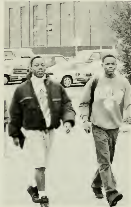
Heading for campus, Nick Cooper and Brandon Cole pass the gym construction site.
