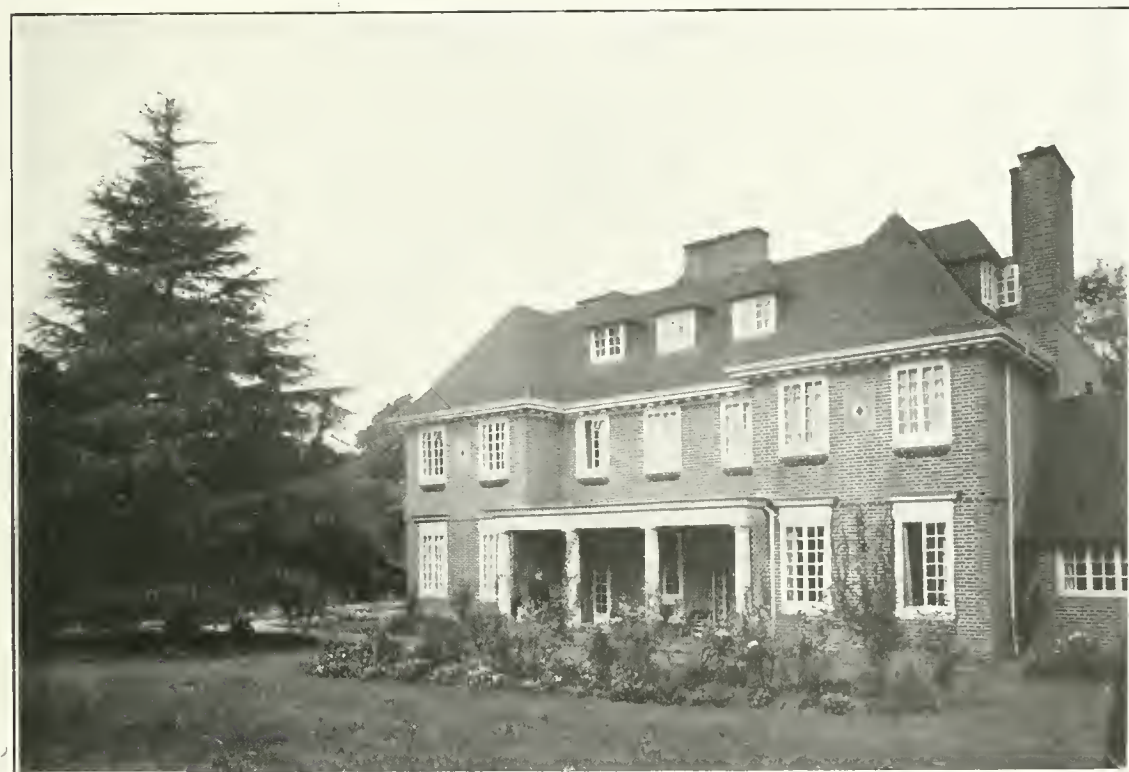
This house is built in the highest part of Camberley, and has fine views from the upper windows. It lies off the main London road between Bagshot and Frimley. Elevations are of red brick, window frames of wood brought out one inch from face of wall. Entrance doorway and columns to loggia in Monk's Park stone.
