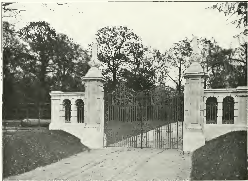
The top view shows the archway and balustrade to the forecourt ; the bottom view, the wrought-iron gates on the drive at the entrance to the garden.
