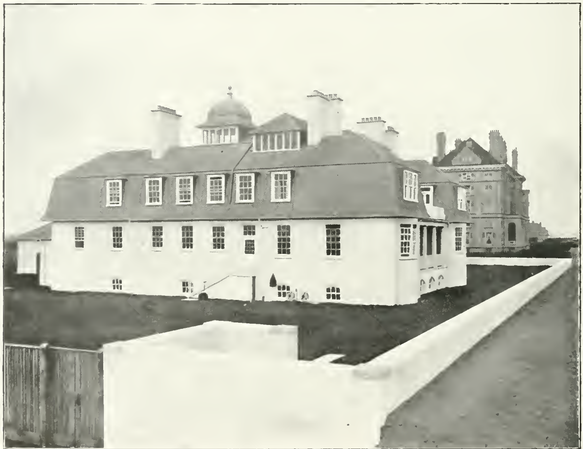
This house is built on the edge of the shore between the Deal and Sandwich Golf Links, and the sea water penetrated within 2 ft. of the footings at high tide.
