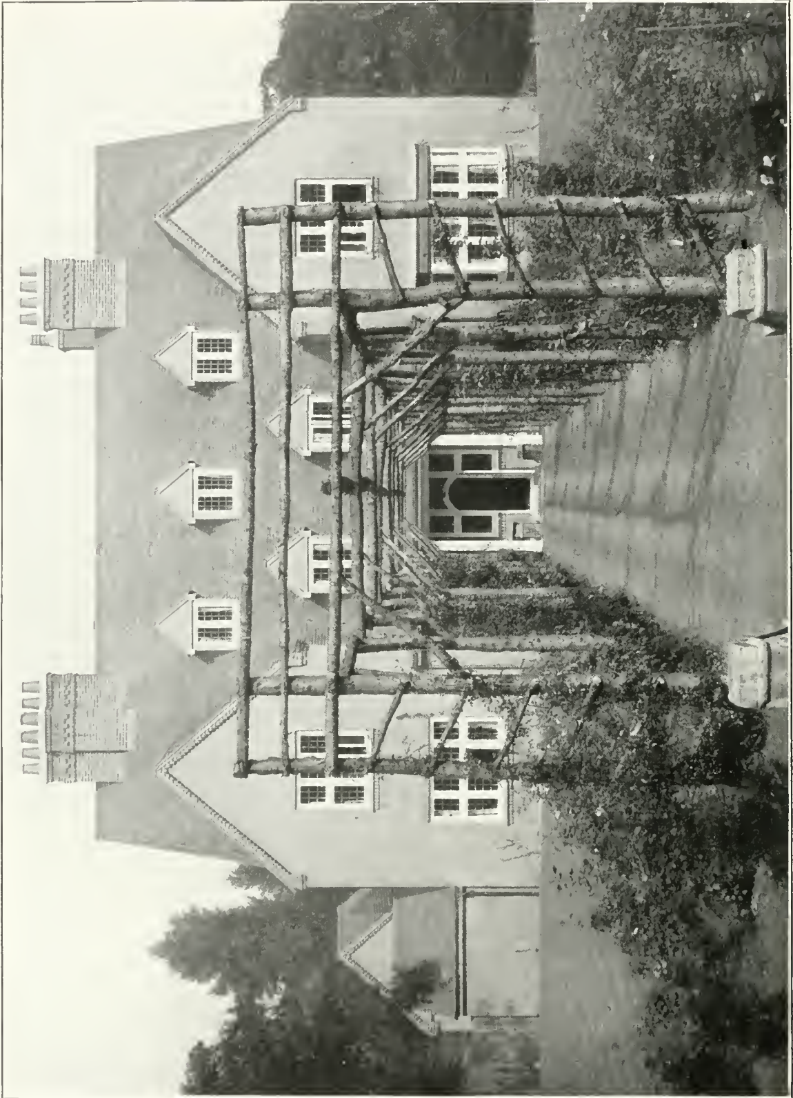
This house is built of stock brick, covered with cement rough-cast left the natural colour. The roofs are covered with hand-made tiles. The windows have wooden casements with leaded lights.
