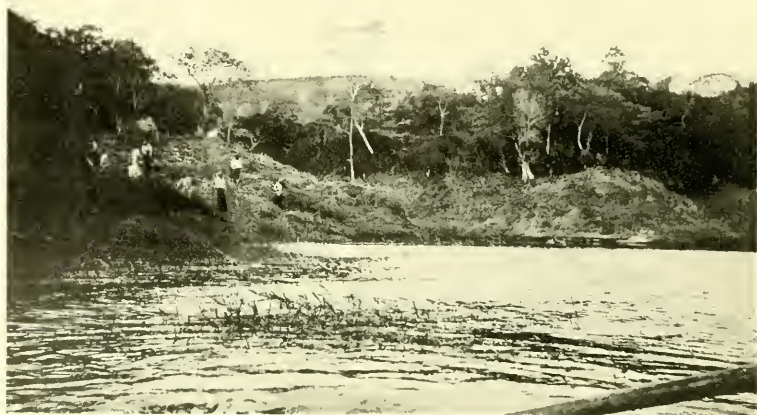
FIG. 79.—Rio Grande Reservoir, Canal Zone, showing workmen clearing the shores to prevent decaying vegetation from falling into the water. This is an old reservoir dating from the time of the French occupation. Photograph by Marsh.
