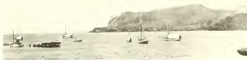
FIG. 75.—Porto Bello Bay, showing excavation in the mountain, where the rock used for the Gatun Dam was secured. Photograph by Busck.
