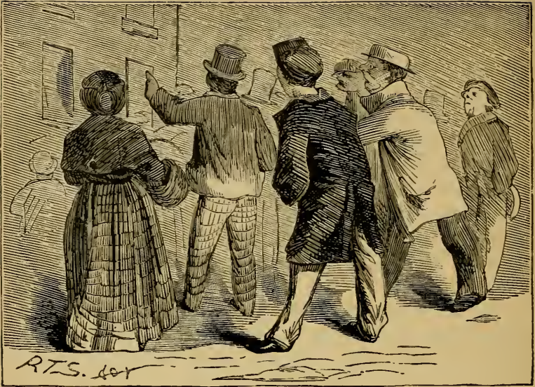
EFFECTS OF AN EARTHQUAKE
