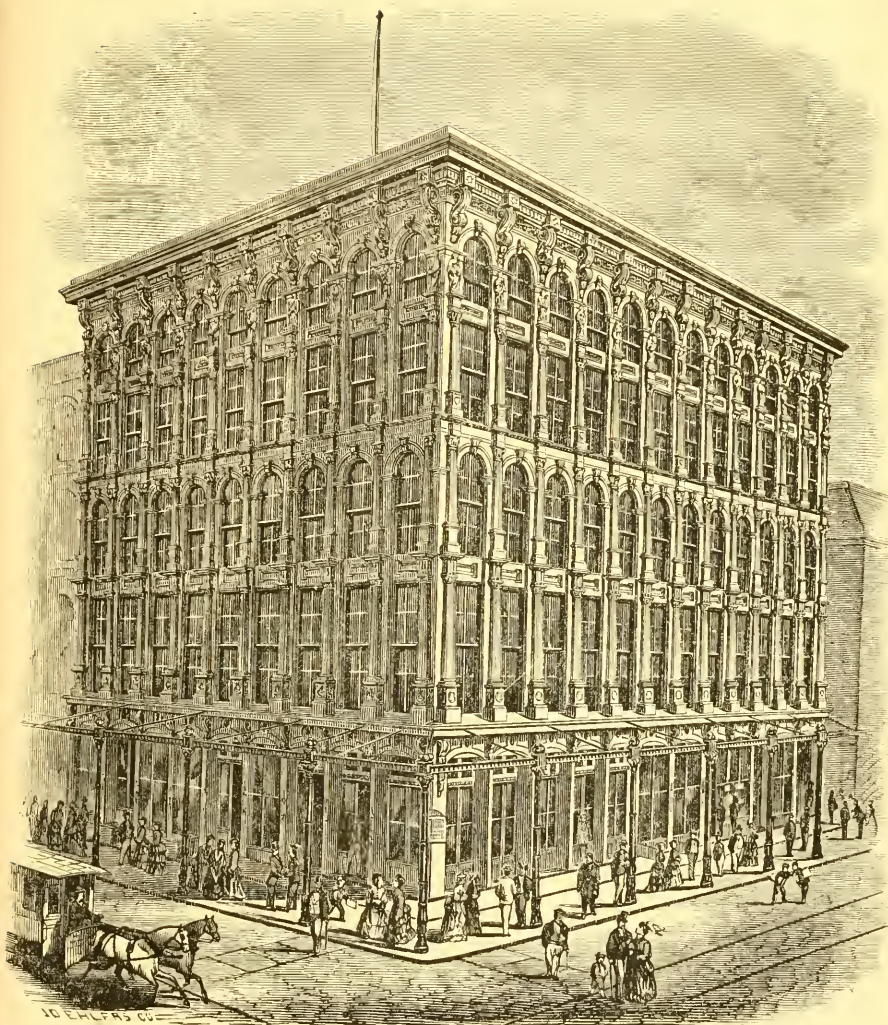
THE "SUN" IRON BUILDING, SOUTHEAST CORNER BALTIMORE AND SOUTH STREETS.
