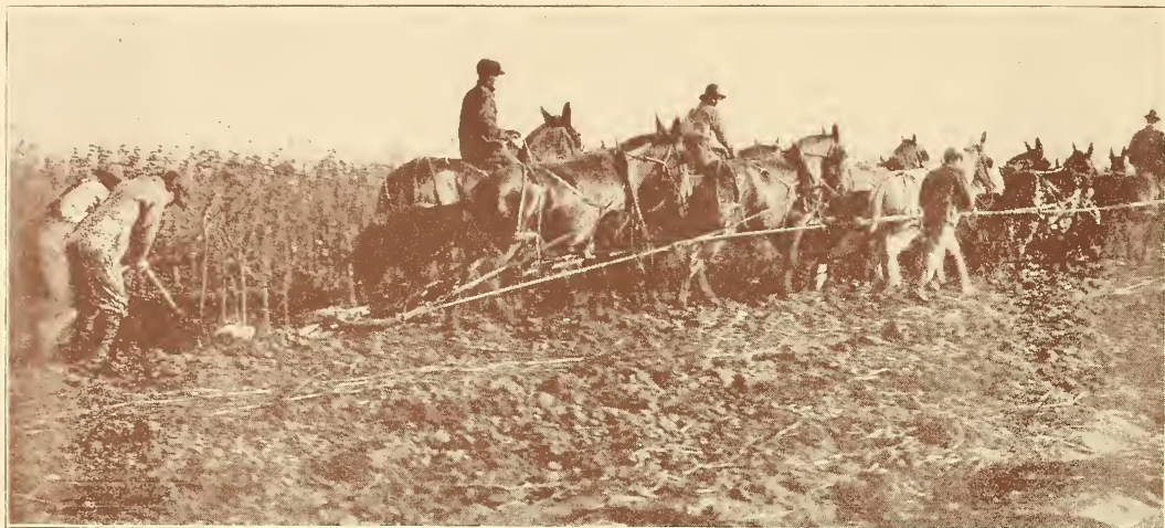
Digging trees with modern digger. You get all the roots
