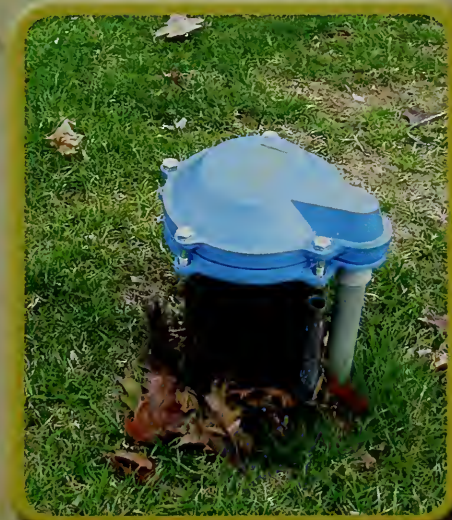
Well owners can protect their drinking water by making sure their well is properly constructed and protected with a well cap. (Photo credit: Stephanie Clemens)
