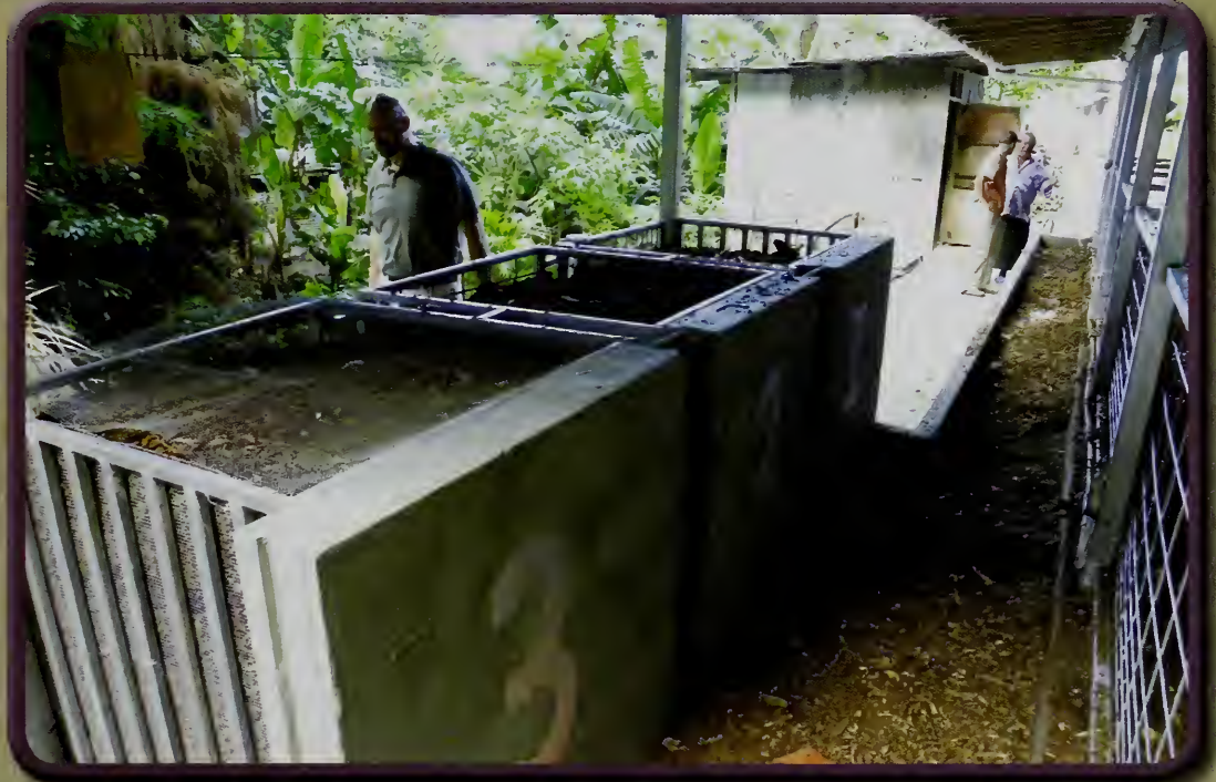
Closing the cycle. The integrated composting system is an important design element of the dry litter technology.
