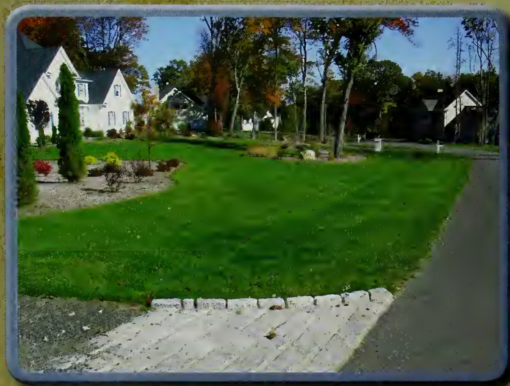
Low Impact Development (LID) practices such as this engineered grassed road swale in Old Saybrook, CT, help promote infiltration of stormwater and reduce runoff. LID is a focus area of the National NEMO Network.
