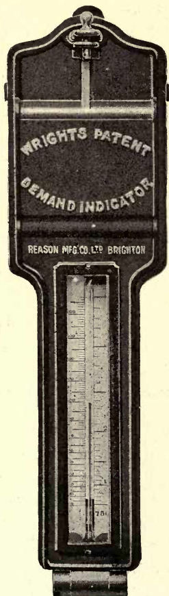
Fig. 246.—Wright's Demand Indicator (Door shut)
