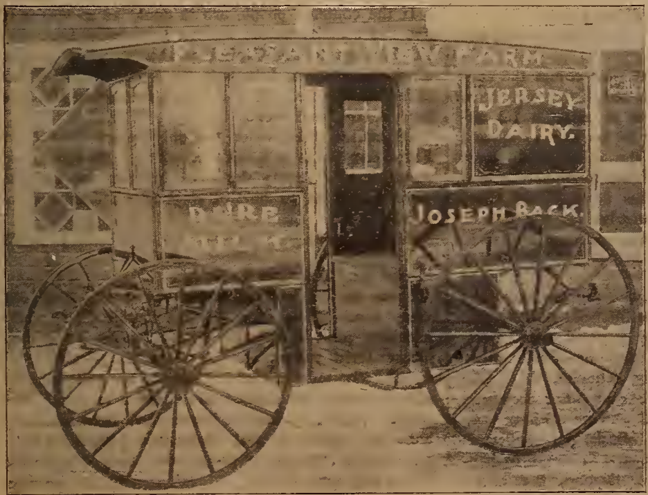
The New Way
