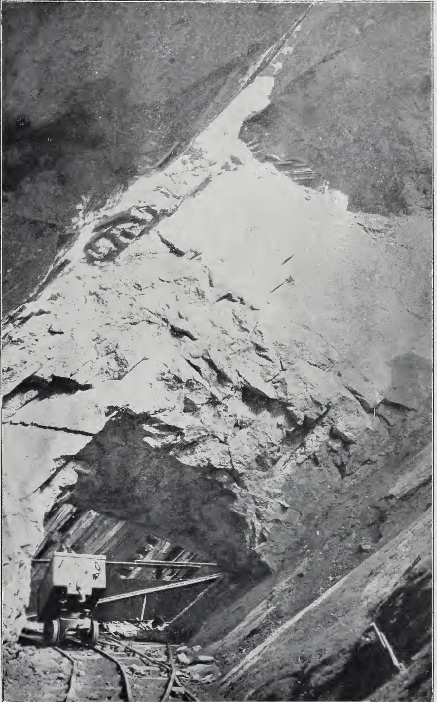
100-foot level at mine of Globe Graphite Mining and Refining Company, concession VI, lot 21, township of North Elmsley, Ont. The pillar indicates the thickness of the ore-body in the east workings.
