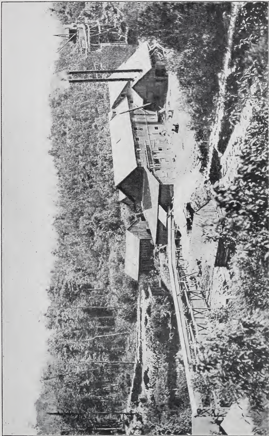
Mill of the Buckingham Graphite Company (North American mine), township of Buckingham, Que. The photograph was taken some years ago, and the buildings are now in a dilapidated condition. The strike of the ore-body is indicated by the tramway, and the main drift enters the mill to the left of the kiln.
