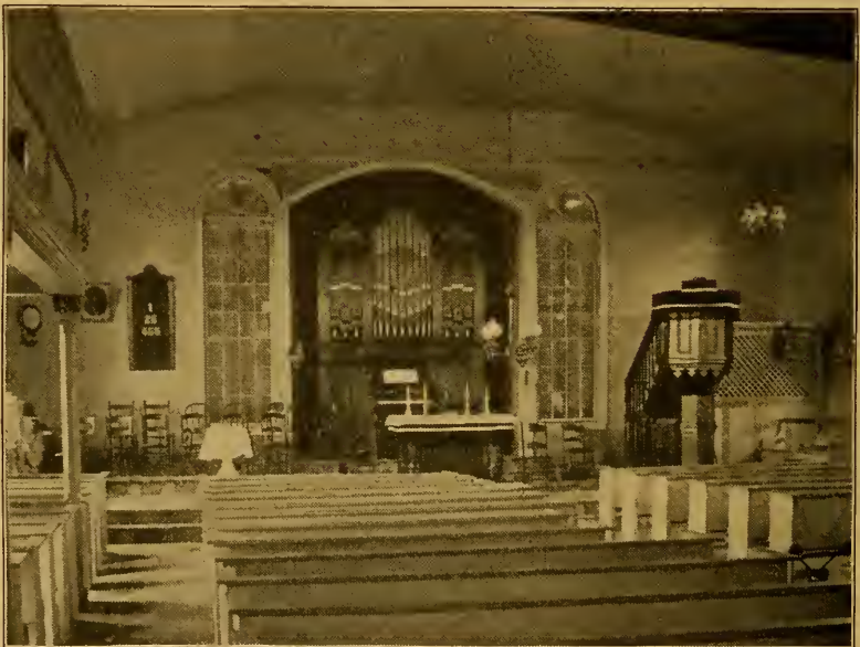
Haysville Church. Interior View.
