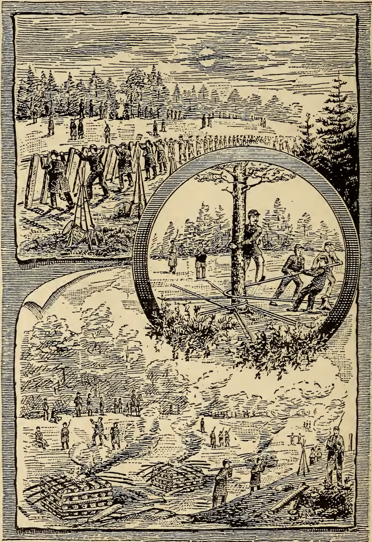
TEARING UP THE WELDON RAILROAD.
