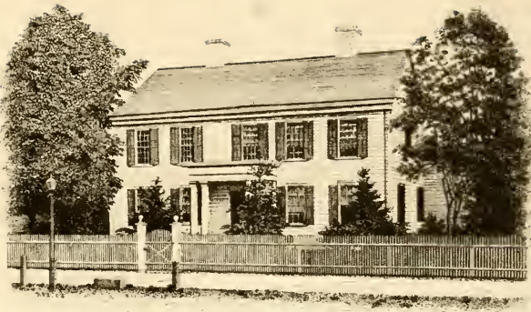
THE PICKERING-ROSS HOUSE, SOUTH MAIN STREET, WILKES-BARRE'
