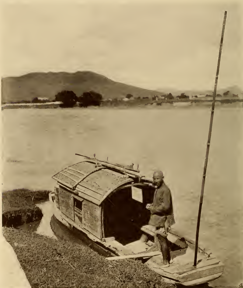
FIG. 44.—A sampan at Shiuchow. This is the common type of small boat used on the rivers of south China. The bamboo pole is used to push the boat in shallow water. Oars are used in deeper water.
