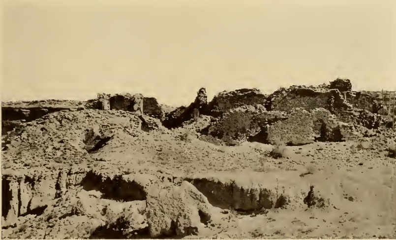
FIG. 118.—Pueblo del Arroyo, occupying an insecure position on the very edge of Chaco wash, 300 feet west of Pueblo Bonito. Flood waters have exposed the remains of an older dwelling beneath the walls of the larger structure and now threaten the latter. View from the north.
