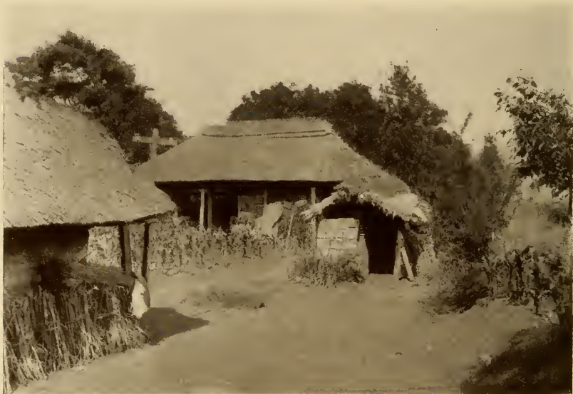
FIG. 34.—A peasant's hut near Gotemba, Japan. The roofs of the building are thatched with coarse grass. The bundles are for firewood.
