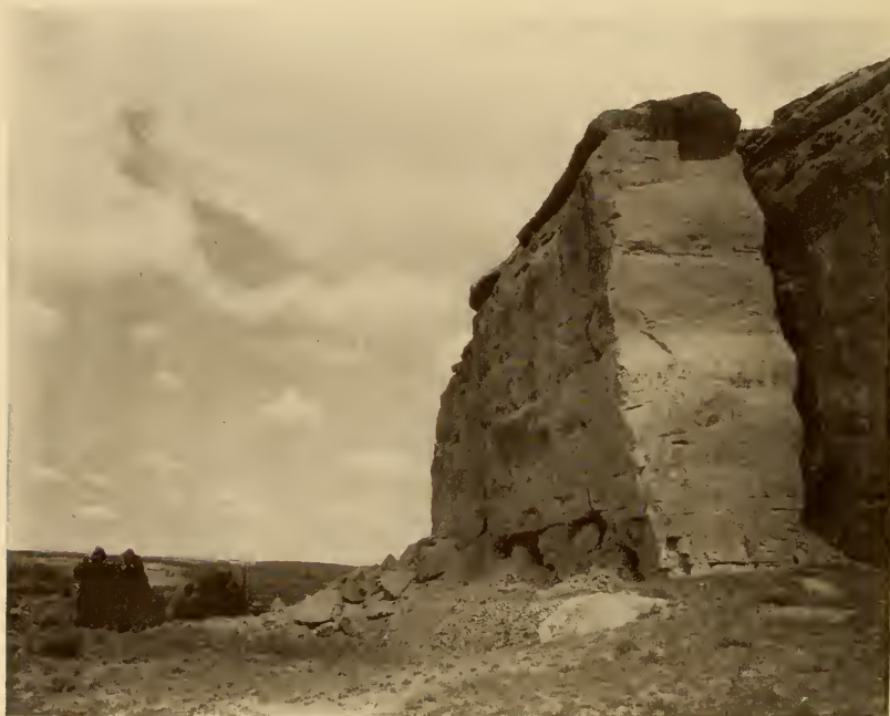
FIG. 121.—A naïve example of Bonitian engineering. In an obvious attempt to hold up a huge section of cliff which threatened to topple upon their village, the ancients placed pine props under the weathered section and covered these with a great terraced mass of masonry. The north wall of Pueblo Bonito stands at the left. (Photograph by Charles Martin. Courtesy of the National Geographic Society.)
