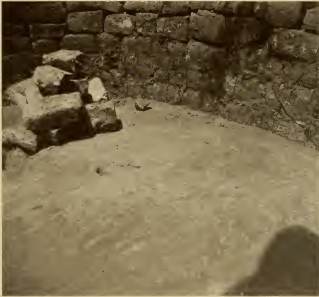
FIG. 107.—Section of floor of Cedar Tree Tower, showing ceremonial opening. Photograph by J. A. Jeancon.
