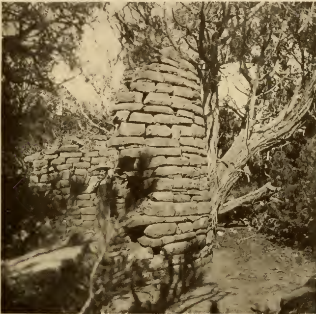
FIG. 104.—Cedar Tree Tower before excavation. Photograph by J. A. Jeancon.
