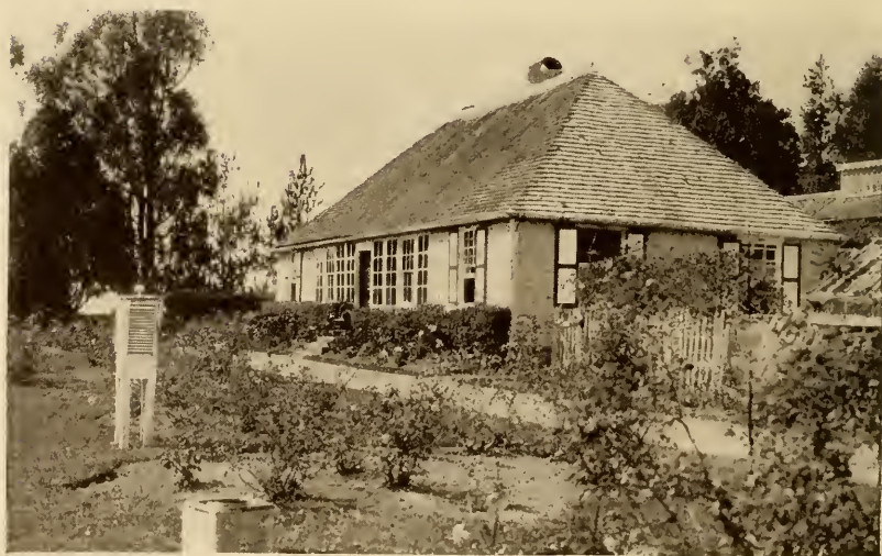
FIG. 62.—Residence at Cinchona.
