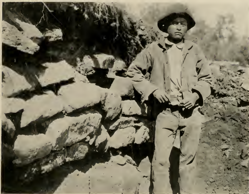
FIG. 66.—Retaining wall of ancient pueblo at Grasshopper Valley, Arizona.
