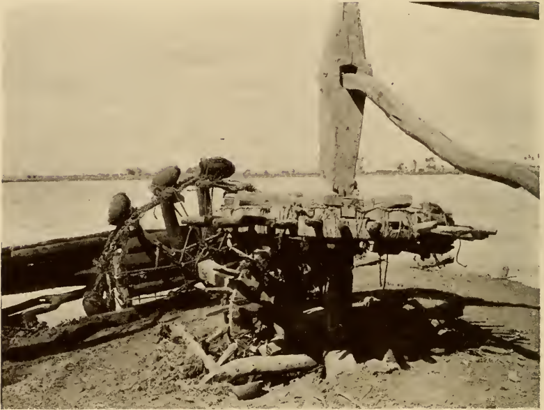
FIG. 42.—Primitive irrigating machinery, on the Blue Nile at Khartoum, August, 1920. Oxen, donkeys or camels are used to turn such water wheels.
