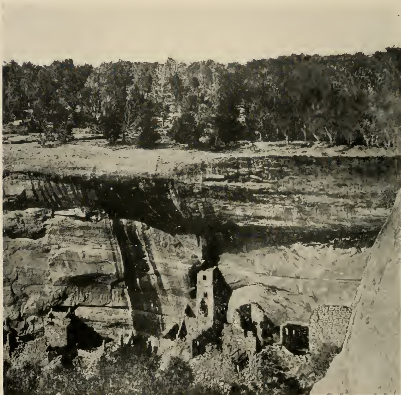
FIG. 49.—Square Tower House before excavation and repair, from Canyon rim.
