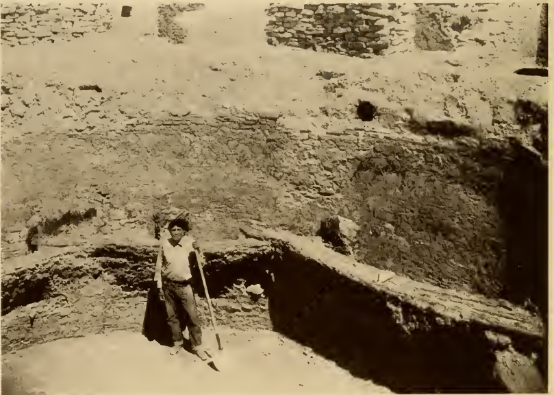
FIG. 113.—An excavated kiva in Pueblo Bonito, showing the low encircling bench and, above this, the roofing timbers which overlap above the pilasters. At the left will be seen the decayed fragments of upright hewn planks which stood between the dome-shaped roof and the circular wall of the chamber. (Photograph by O. C. Havens. Courtesy of the National Geographic Society.)
