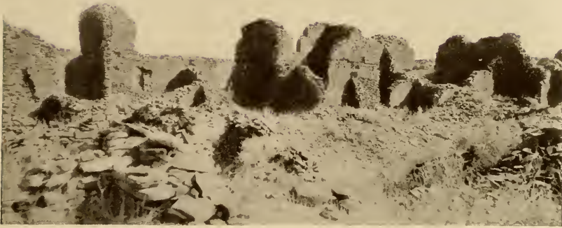
FIG. 117.—A portion of Kimmenioli ruin, showing the present condition of its walls. About 135 ground floor rooms are still traceable; originally the building was three, perhaps four, stories high. Although one of the finest in the national monument this great communal dwelling is not so well known as some of its neighbors in Chaco Canyon which is situated some ten miles to the north and east.
