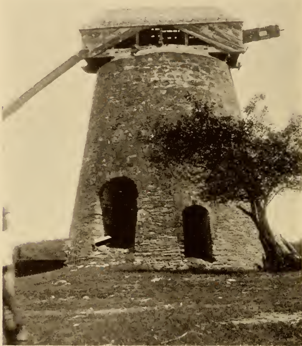
FIG. 68.—Antigua. An old sugar mill. These old stone mills, formerly used for crushing the cane, are common on the islands. Oxen were attached to the long beam. The crushing or grinding is now done in modern sugar factories.
