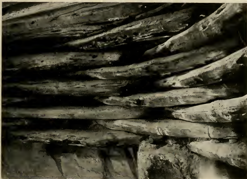
FIG. 53.—View from below of one sector of original roof logs of kiva 'A'. Photograph by Gordon Parker.
