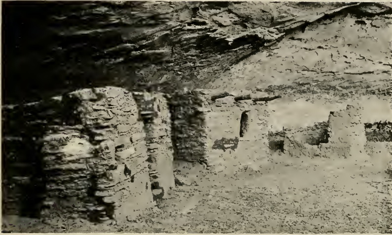
FIG. 68.—Isolated rooms forming part of a small cliff village in Cottonwood Canyon. Several of the rooms were repaired after excavation; the darker portions show the extent of these restorations.
