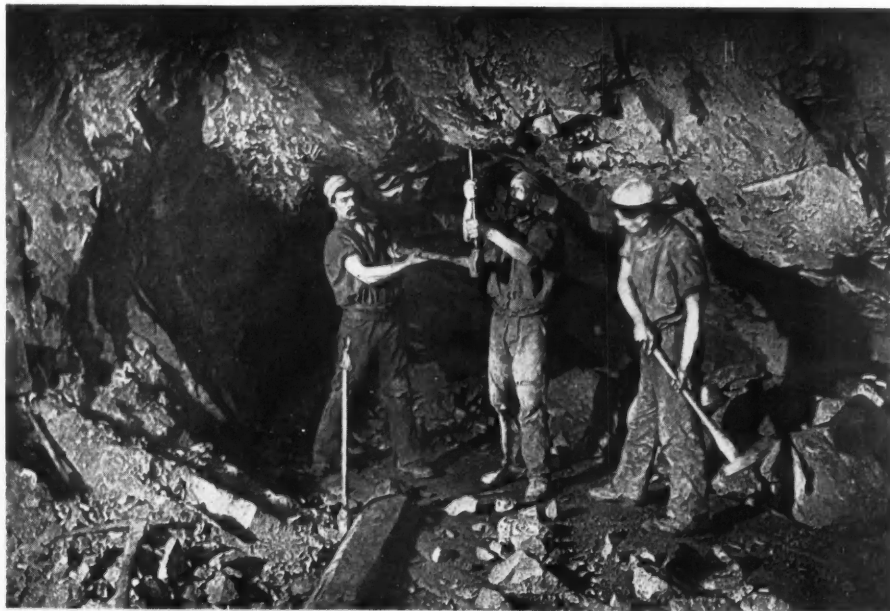
12. BORING AN UPPER, EAST POOL MINE.
