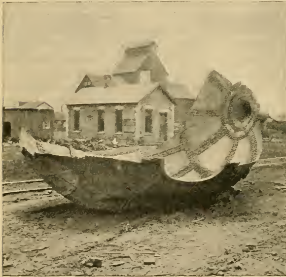
FIG. 2.—AN EXPLODED ROTARY.
