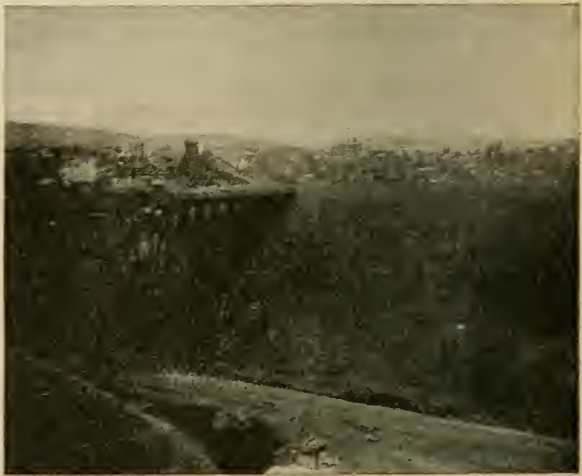
FIG. 4.—RAILROAD BRIDGE BETWEEN CULM PILES.
