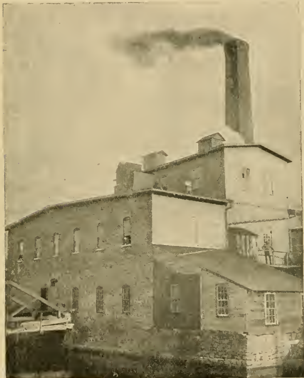
FIG. 3.—THE BUILDING THAT CONTAINED THE ROTARY IN FIG. 2. (BEFORE THE EXPLOSION.)
