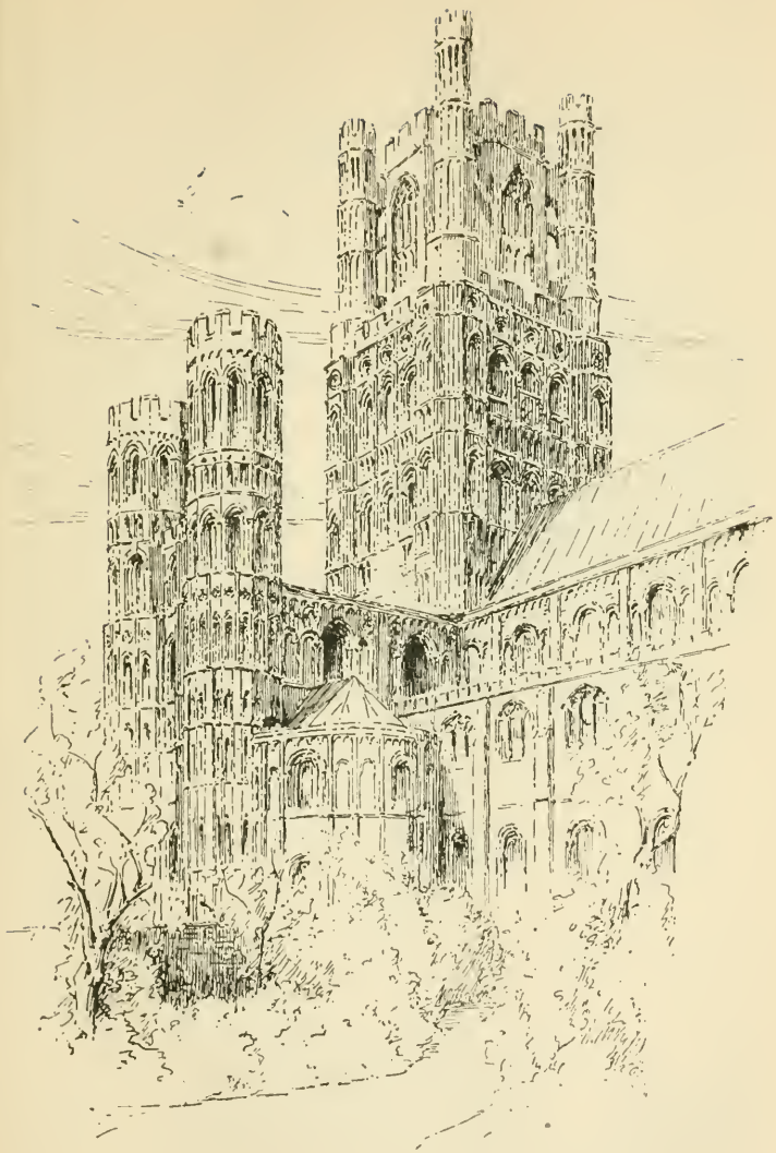
WEST TOWER FROM DEANERY GARDENS
