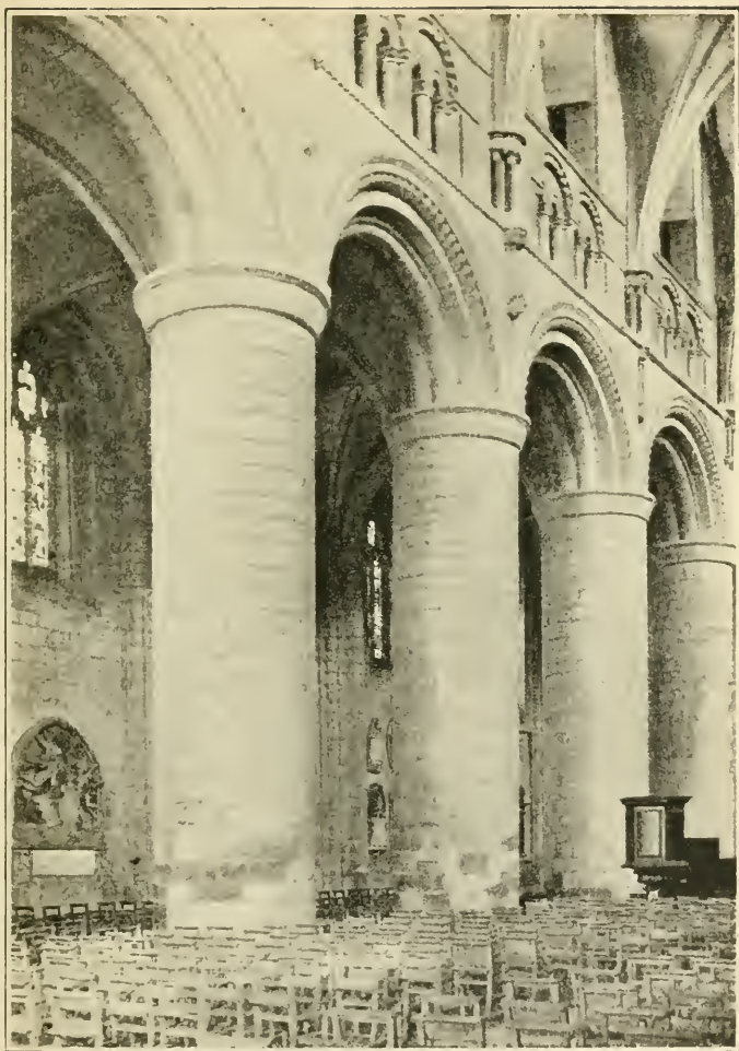
NAVE PILLARS FROM THE WEST
