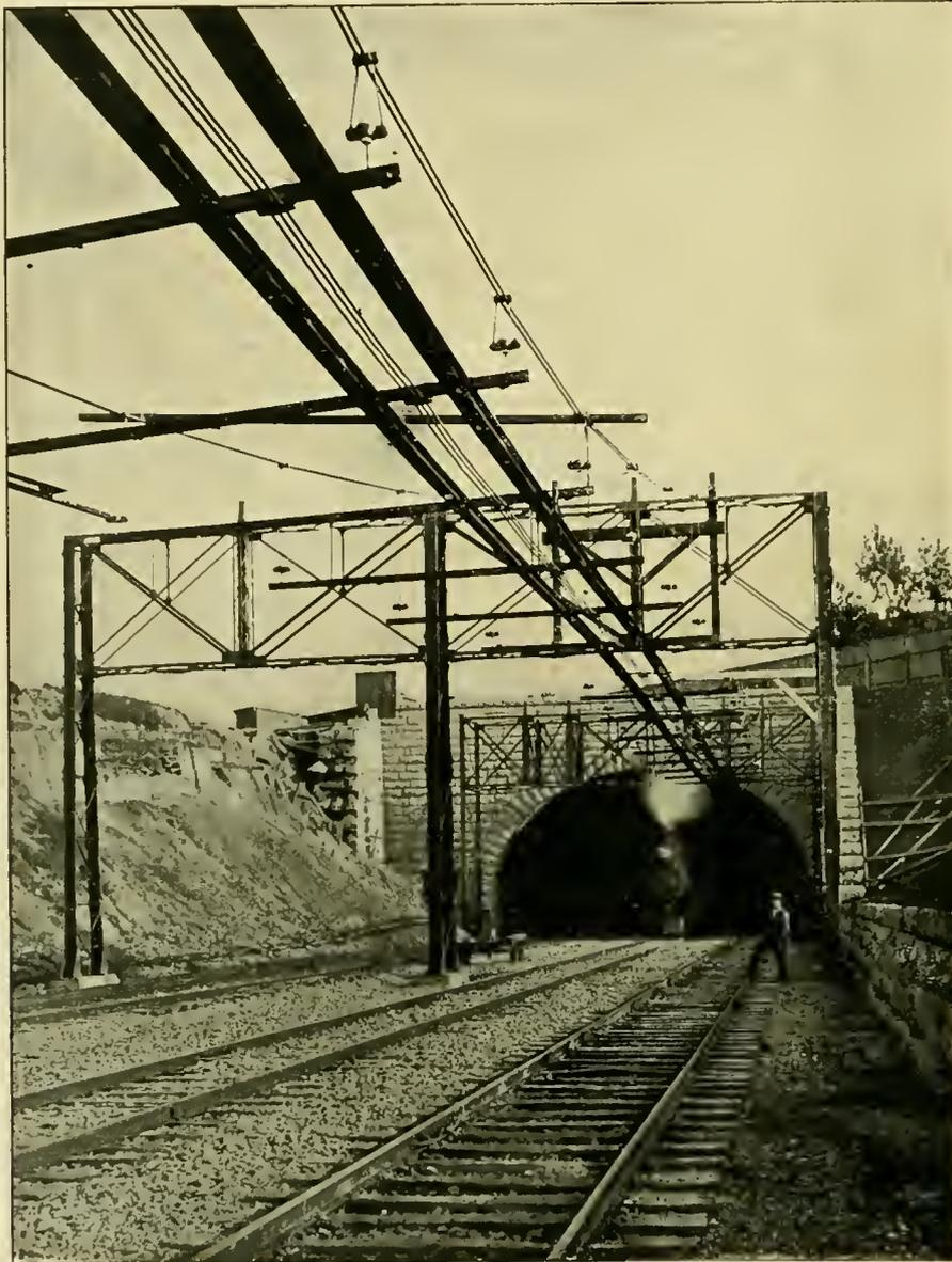
OVERHEAD CONSTRUCTION AT ENTRANCE TO TUNNEL.
