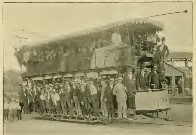
built from designs by Mr. Harrison, is mounted on a Peckham truck and driven by two 30-horse-power Walker motors. By no means the least interesting feature of the load was the Sterling fare register which showed 175 fares—the number of passengers carried at one time on this trip.
