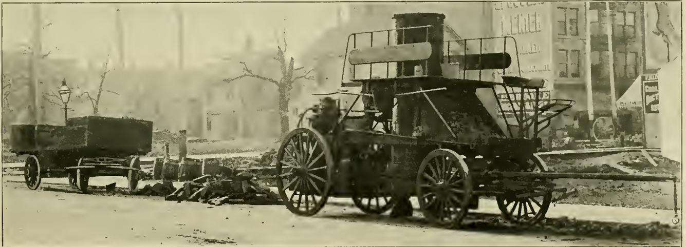
CUPOLA AND SUPPLY TRUCK FOR CAST WELDING JOINTS, 1895 PATTERN.
