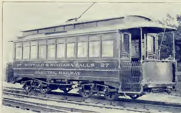
MOTOR CAR—MOTOR ON EACH AXLE.
