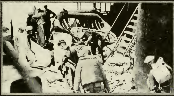
SORTING THE DEBRIS
