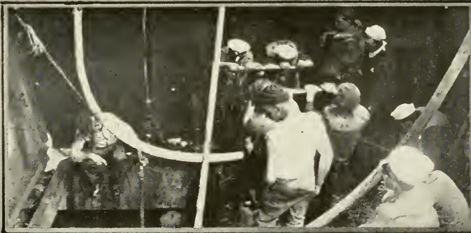
ANOTHER VIEW OF THE PUMPS
