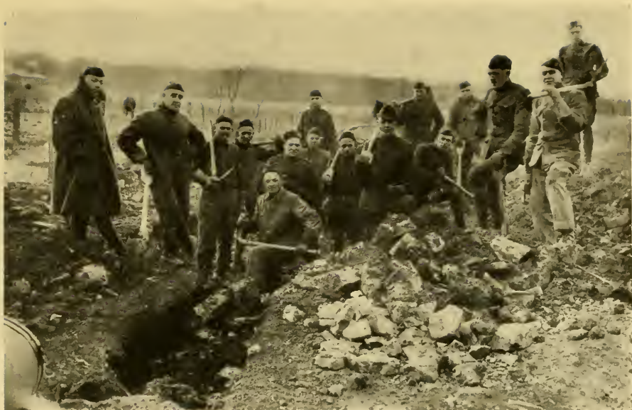
DETAIL INSTALLING TANK AT GARAGE
