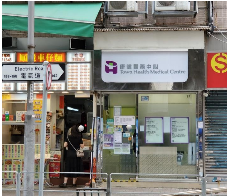
Shop front of the Medical Centre
