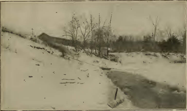
SHOWING CREAMERY WATER SUPPLY, NARROWSBURG.
