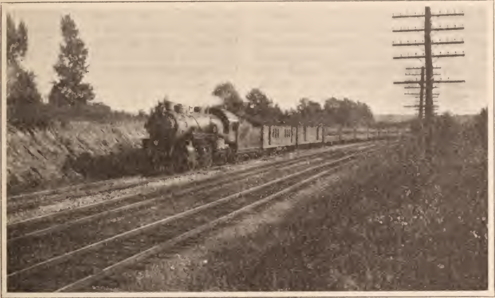
HEAVY PASSENGER TRAIN MOVING ON SCHEDULE TIME ON AN UP-GRADE WITHIN LIMITS OF DISTRICT OF COLUMBIA—AND WITHOUT SMOKE
