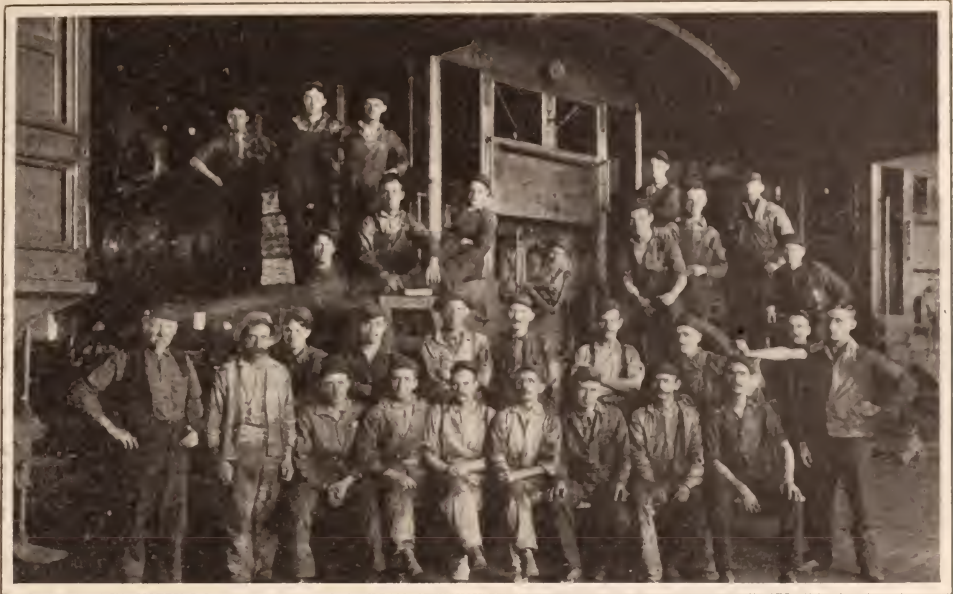
NEWARK, OHIO, ERECTING SHOP FORCE IN 1909
