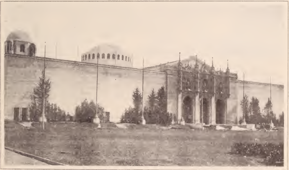
THE GREAT PALACE OF TRANSPORTATION AS SEEN FROM THE NORTH GARDENS
