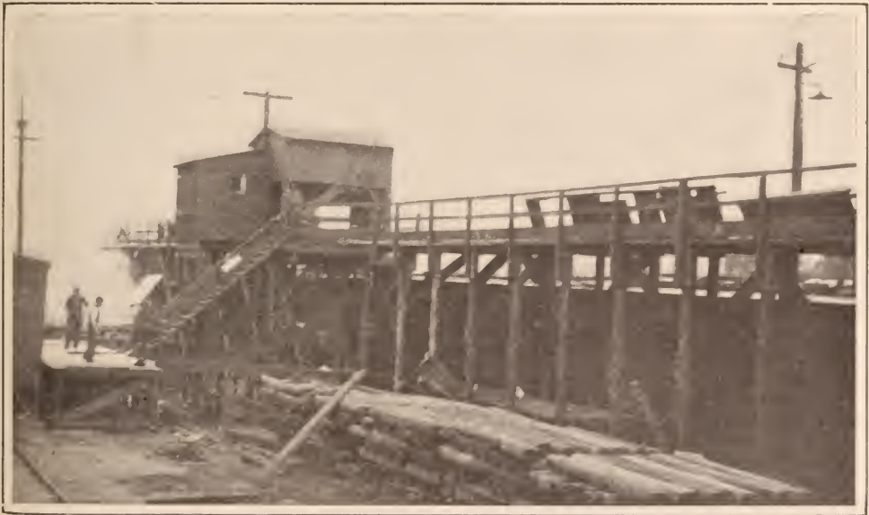
PLATFORM AT CUMBERLAND FOR ICING REFRIGERATORS
