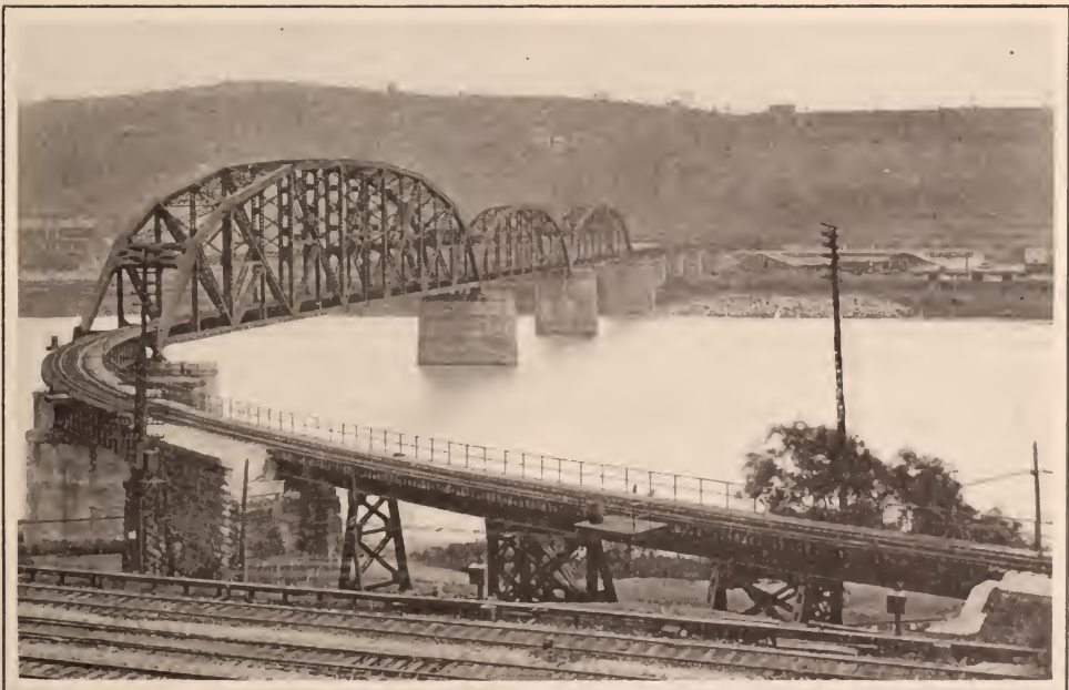
BRIDGE No. 74, W. P. & B. BRANCH over the Monongahela at Wheeling Junction, Pittsburgh Division, showing the recently completed east approach
