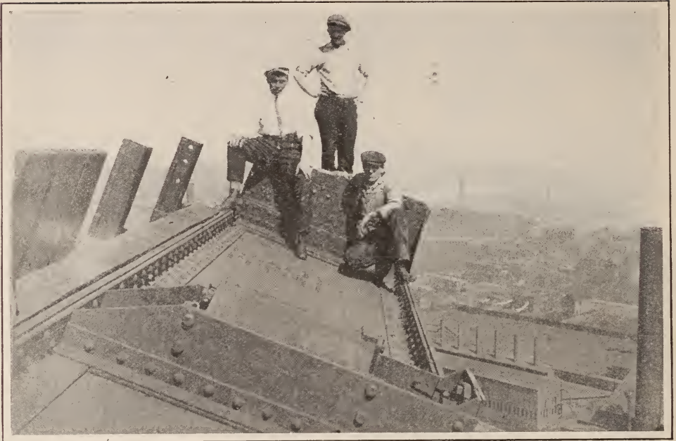
BASCULE BRIDGE AT CHICAGO
