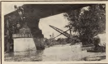
COUPLING UP THE NEW SPAN
