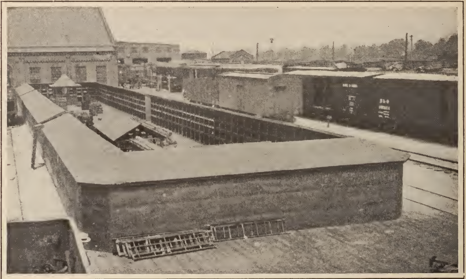
PLATFORM AND BINS 34 x 210 FEET, BUILT AT KEYSER FOR STORING CAR MATERIAL Constructed entirely from second-hand lumber obtained from dismantled freight cars
