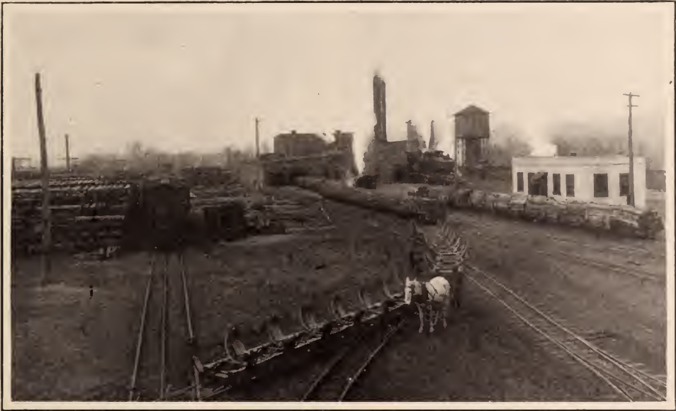
GENERAL VIEW OF TIMBER TREATING PLANT AT GREEN SPRING, W. VA.
