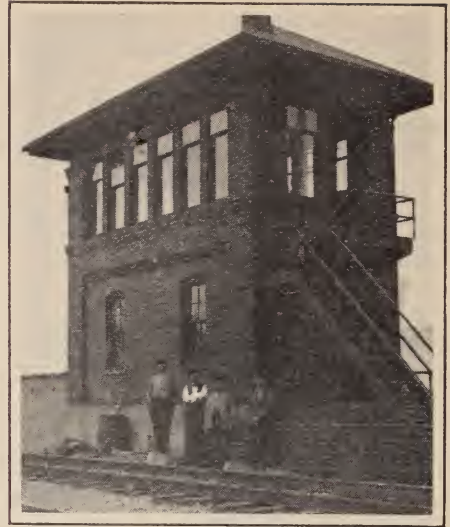
OPERATING TOWER AT THE BRIDGE
