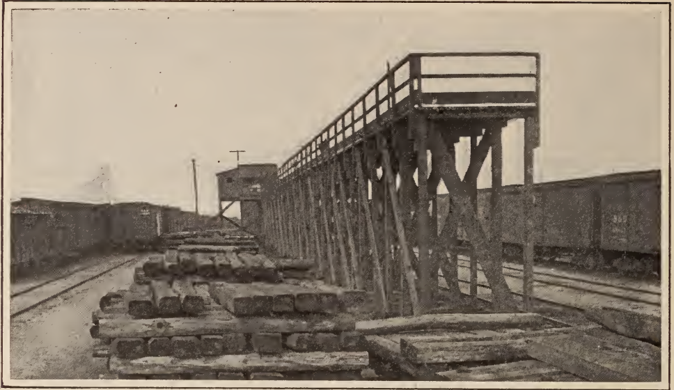
NEW ICING PLATFORM AT CUMBERLAND
