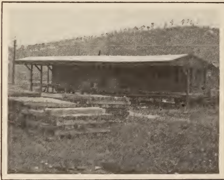
FRUIT LOADING PLATFORM 90 FEET LONG Built at Keyser entirely from second-hand material, most of which was obtained from dismantled cars
