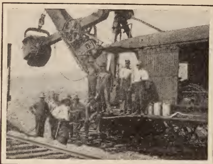
FOREMAN A. GROMBAUGH AND CREW AT HAMILTON GRAVEL PIT
