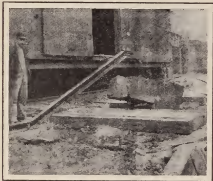
WHAT POOR TRAIN HANDLING DOES TO YARD EQUIPMENT AND—
