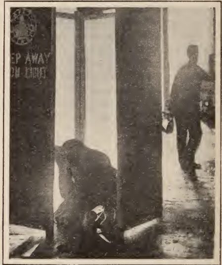
SCREEN USED TO PROTECT EYES FROM PIERCING LIGHT OF ELECTRIC WELDER
