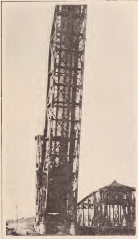
COLOSSAL IN SIZE, THIS BASCULE BRIDGE HAS THE PRECISION OF FINE WATCH WORKS
