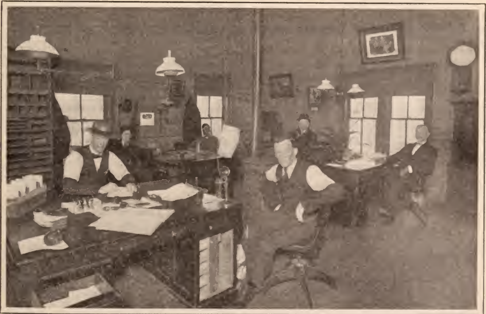
MT. VERNON, OHIO, FREIGHT OFFICE AND FORCE
