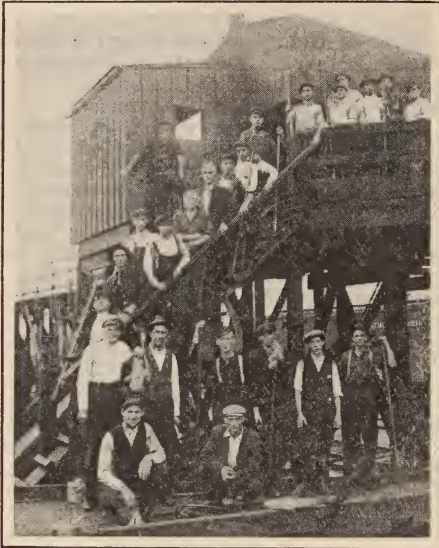
RECORD BREAKING ICING CREW AT CUMBERLAND YARD
