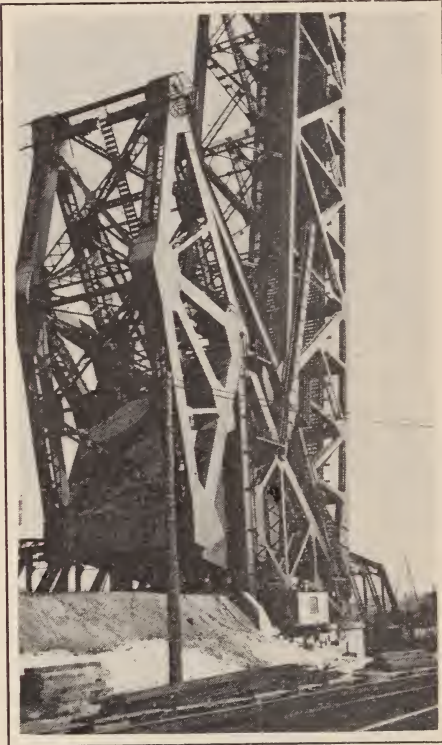
CEMENT BLOCKS BALANCE THE ENORMOUS WEIGHT OF THE BRIDGE
