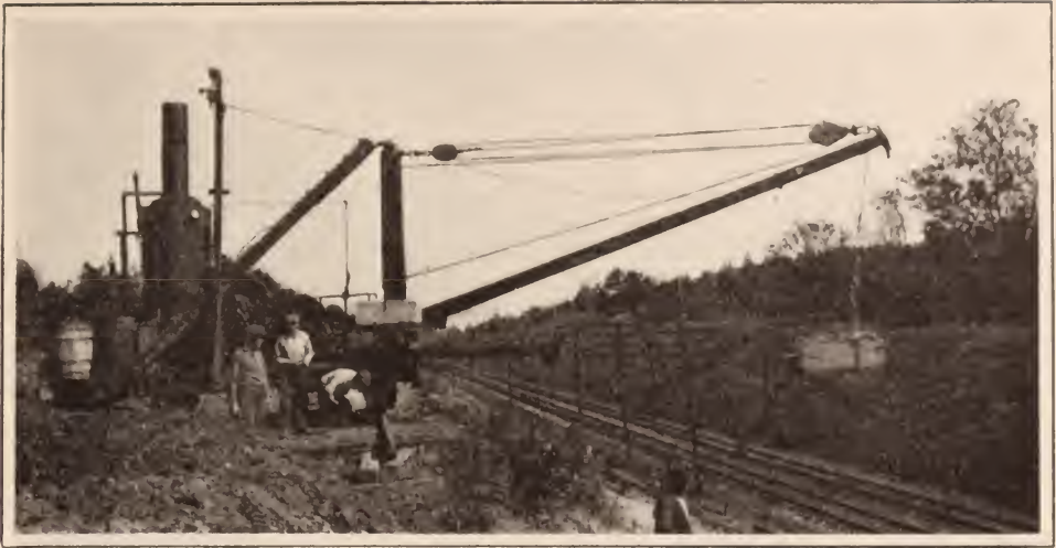
No. 1—STATIONARY ENGINE AND HOISTING ARRANGEMENT
