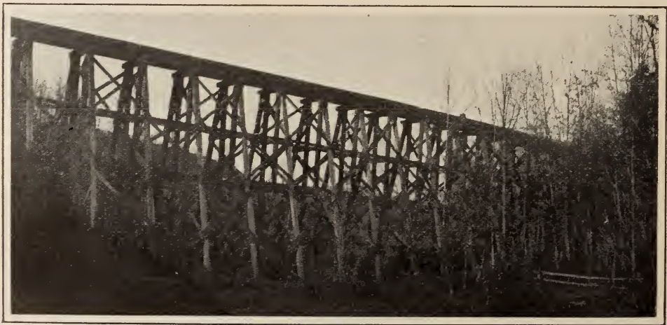
TRESTLE 63, R. S. & G. BRANCH OF THE OHIO RIVER DIVISION
