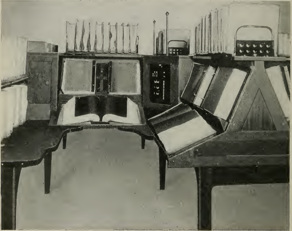
THIS CLOSE-UP of an Information position illustrates desk design to make voluminous records, such as those for a metropolitan area, readily available to the operator
