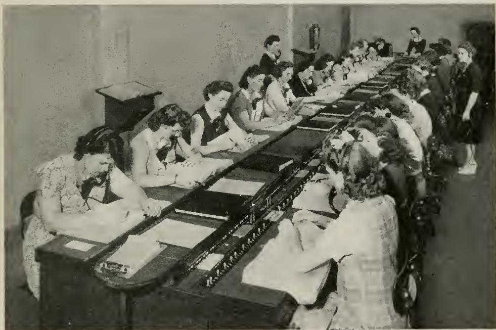
AN EXAMPLE of a modern type of No. 1 Information Desk, equipped with team-work circuits. This type of desk normally provides an average-size team of 12 operators
