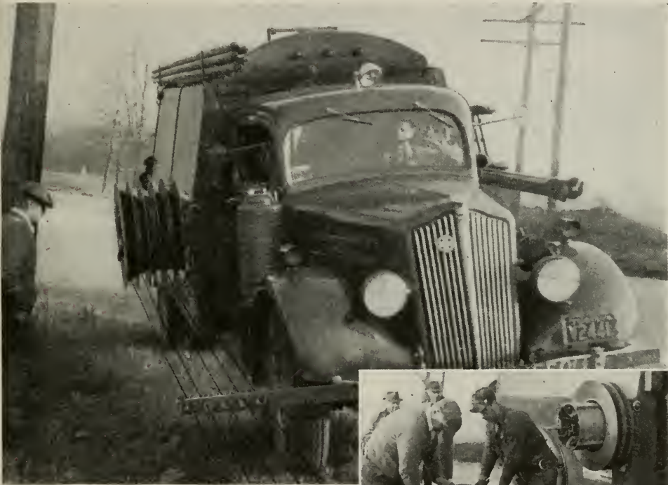
THE SPECIALLY designed take-up reel avoids damage to copper wire during removal. Wires are wound into individual coils
