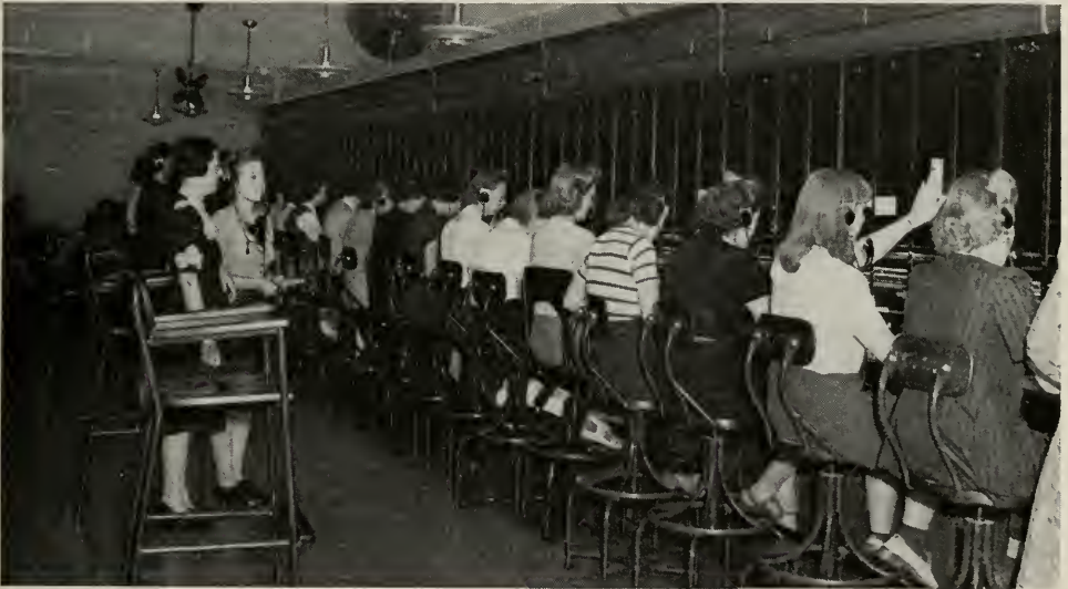
TWO YEARS AGO this long distance switchboard, with its 20 operator positions, did not exist. It was placed in operation to handle the messages for an Army training area
