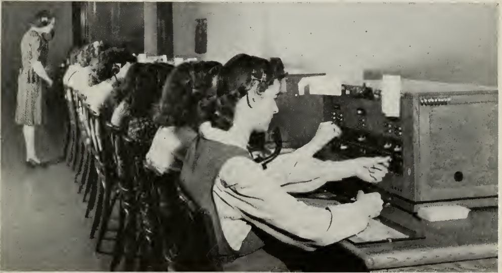
THESE SUPPLEMENTARY CABINETS used for handling long distance calls contain less than one-sixth of the metal in regular switchboard positions—although requiring twice as many operators to handle the same volume of traffic
