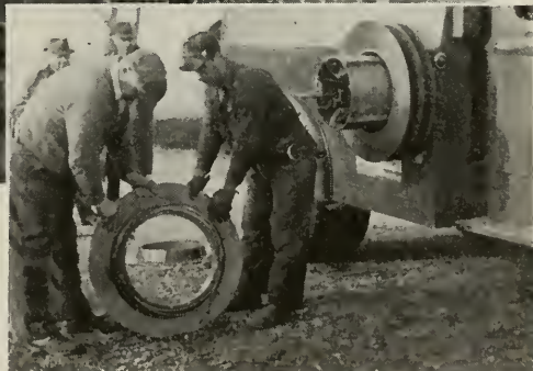
THE SPECIALLY designed take-up reel avoids damage to copper wire during removal. Wires are wound into individual coils
