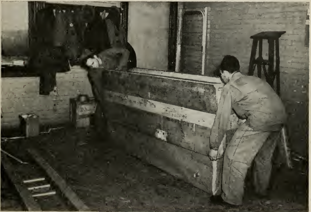
SIGNAL CORPS MEN are removing the packing case from one unit such as is shown on page 243 before up-ending it onto the base which has been prepared at the left to receive it
