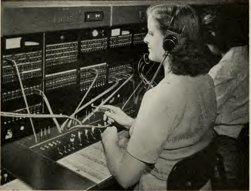
CALLS WHICH could not be completed originally through the No. 4 System because of busy circuits are handled at the No. 5 switchboard
