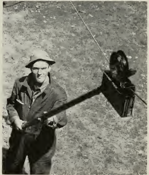
THIS INGENIOUS little contrivance paints drop wires while they are in the air, so that they need not be lowered to the ground
