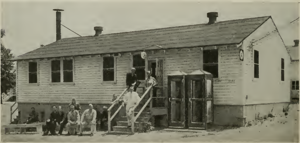
A CAMP TELEPHONE BUILDING. Men waiting on the benches outside are summoned by loud-speaker when their calls are ready. The outdoor booths are for use during hours when attended service is not provided
