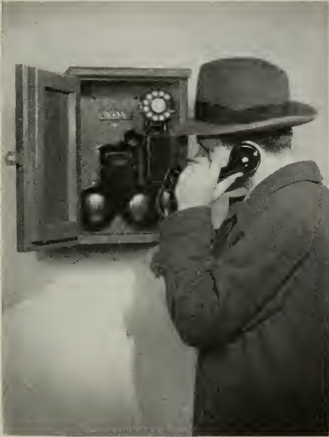
THE HOUSING of the outdoor telephone set is now made of wood instead of metal
