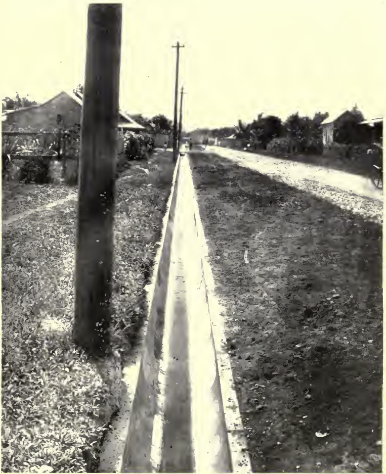
FIG. 20.—A CONCRETE ROADSIDE DRAIN, PORT OF SPAIN, TRINIDAD.
