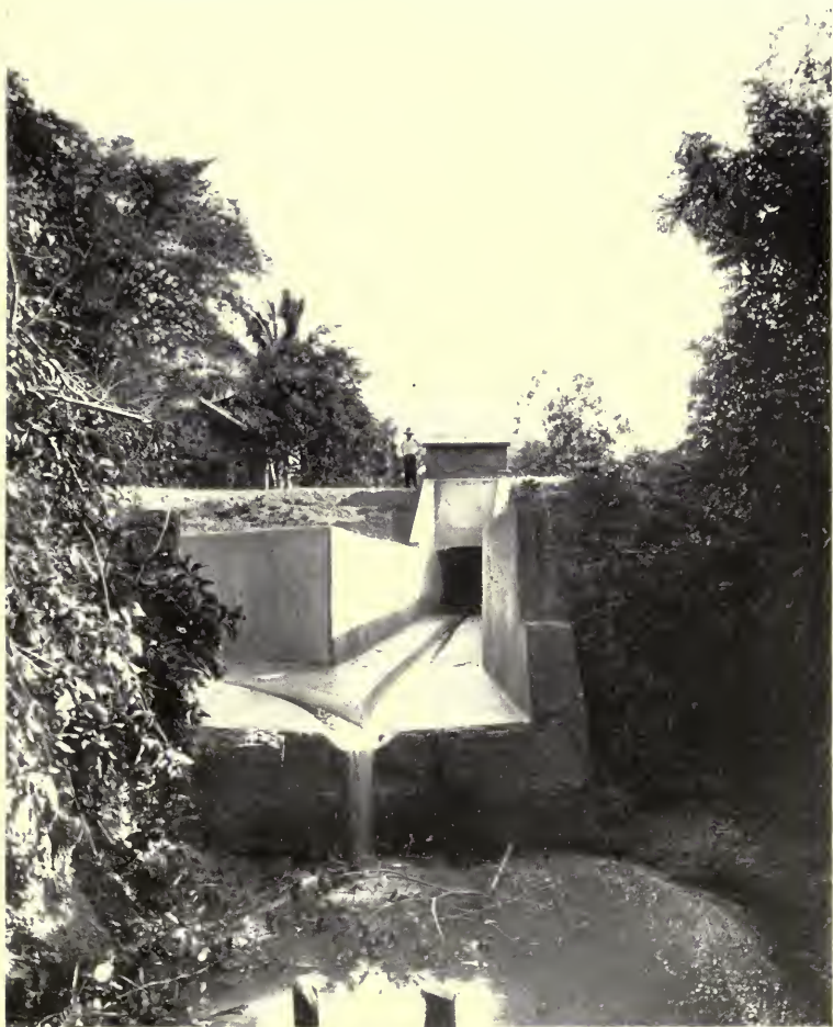
FIG. 28.—LARGE CONCRETE DRAINS, PORT OF SPAIN, TRINIDAD.
