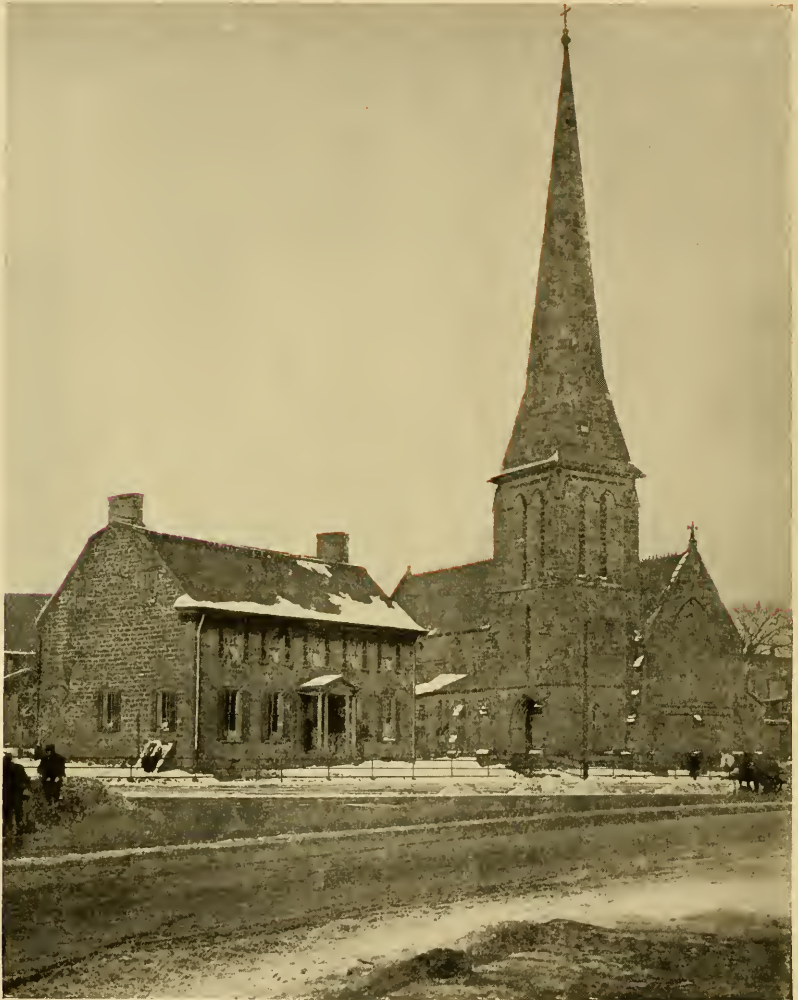
HOUSE OF PRAYER AND PARISH HOUSE
