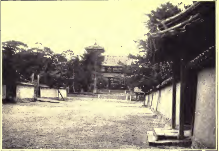
THE OLDEST WOODEN STRUCTURE IN THE WORLD—IIORIJU PAGODA
