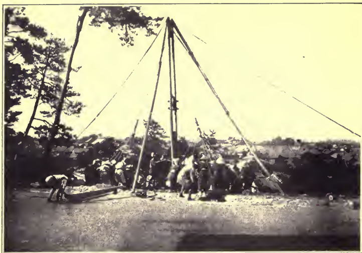
WOMEN PILE-DRIVERS EACH WITH A ROPE-END AND A PATHETIC CHANT
