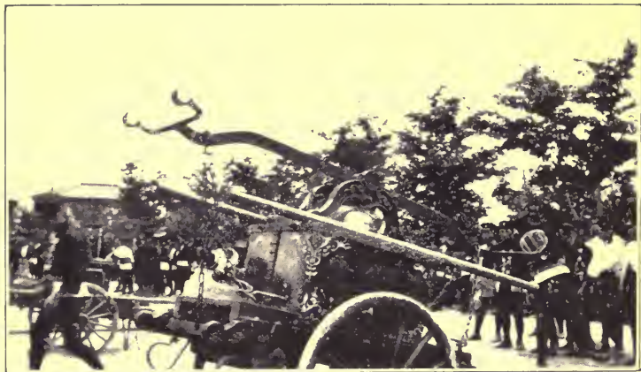
WHILE THIS PUMP PUMPS THE FIRE BURNS
