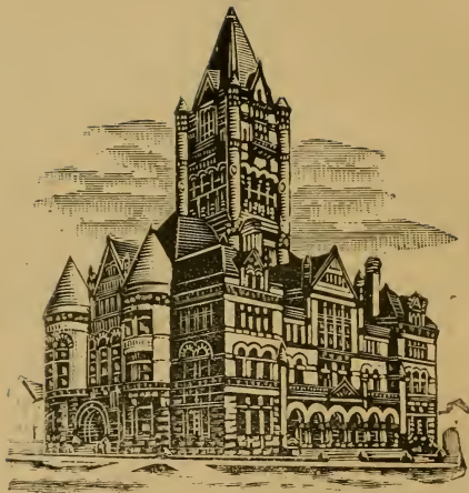
KENT COUNTY COURT HOUSE. Cor. Crescent Avenue and Kent Street.
