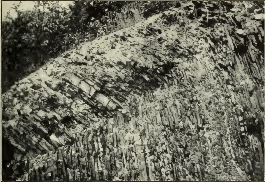
FIG. 1.—VIEW SHOWING BENDING OF ROMNEY SHALE DUE TO CREEP IN CUT OF WESTERN MARYLAND RAILROAD WEST OF TONOLOWAY.
