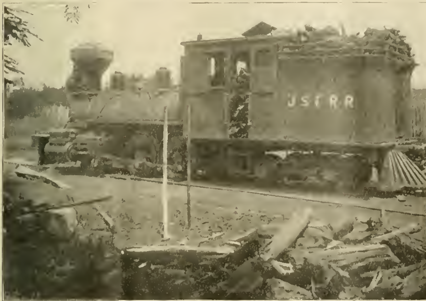
OLD WAR TIME ENGINE NOW ON CONSTRUCTION.
