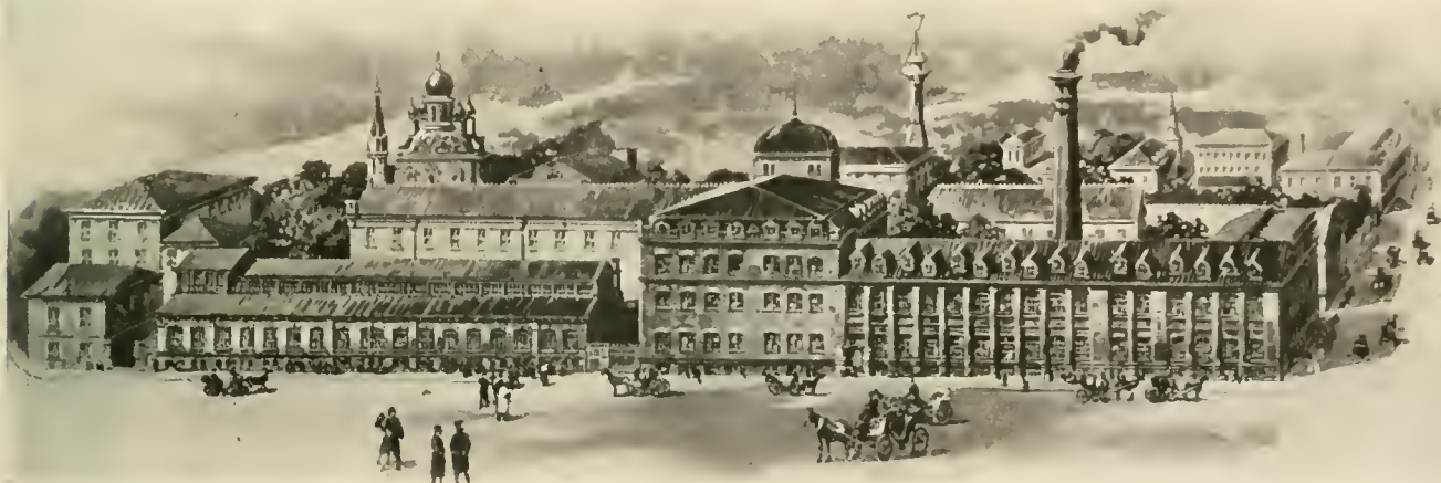
OFFICES AND FACTORY WORKS OF THE WESTINGHOUSE AIR BRAKE COMPANY AT ST. PETERSBURG, RUSSIA.
