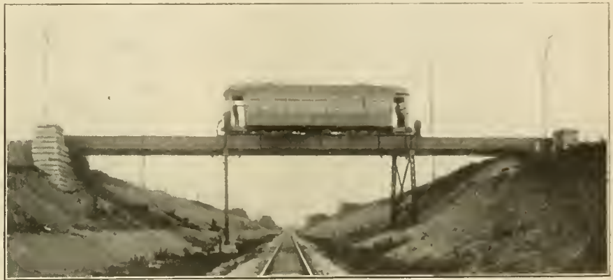
WESTERN OHIO ELECTRIC OVERHEAD CROSSING, C. & E. RAILWAY.
