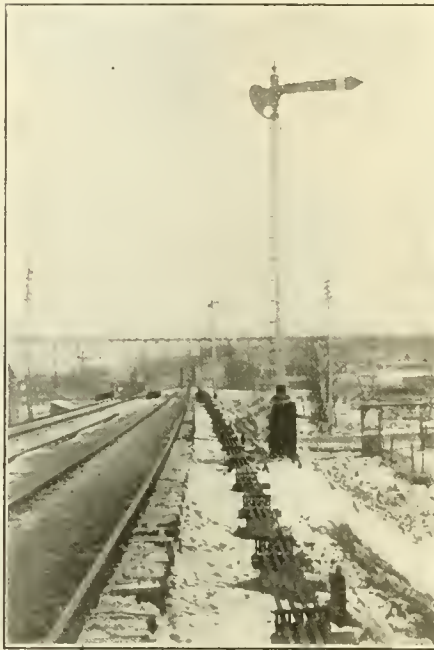
UNION SWITCH AND SIGNAL CO.'S MOTOR DRIVEN AUTOMATIC SIGNAL.
