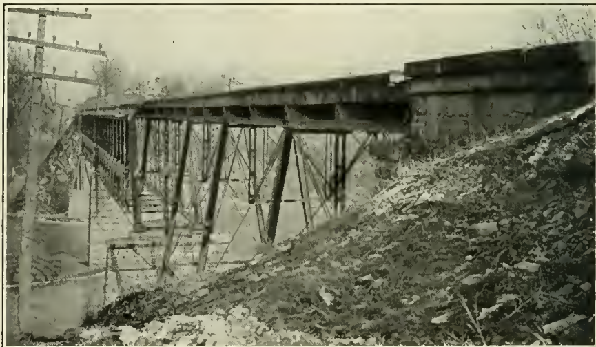
VERMILLION TRESTLE, NICKEL PLATE LINE.
