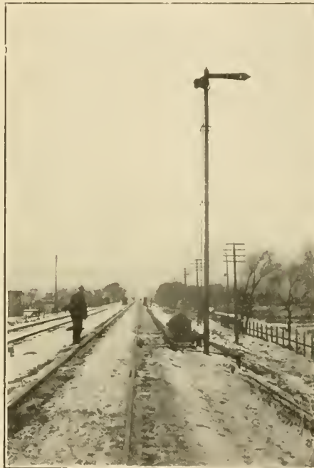
ROWELL-POTTER AUTOMATIC BLOCK SIGNAL.
