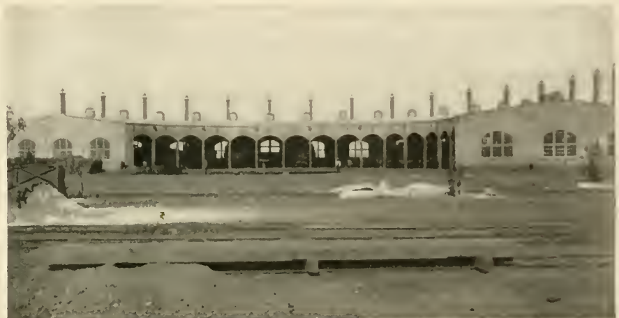
ENGINE HOUSE, MONCLOVA, MEXICO. MEXICAN INTERNATIONAL RAILWAY. GENERAL REPAIR SHOPS TO BE BUILT LATER.
