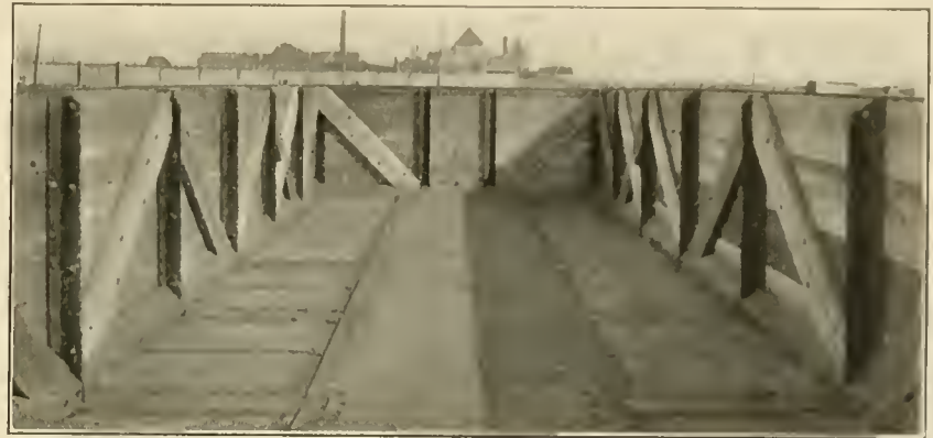
CASWELL DUMP CAR—DROP DOORS CLOSED.
