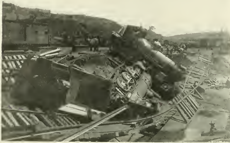
FIG. 3. THE "SANTA FE SINK HOLE."
