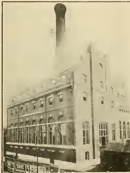
POWER HOUSE—BOSTON ELEVATED.
