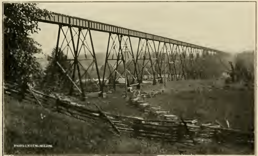
TRESTLE ON NICKEL PLATE LINE.
