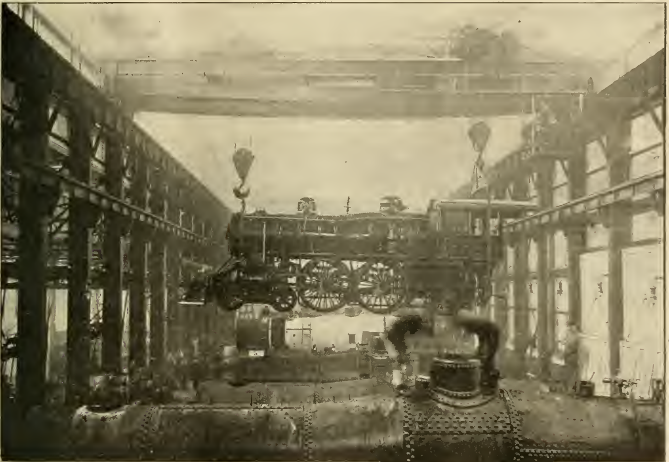
ROGERS ERECTING SHOP.—BIG C., B. & Q. ENGINE HANGING IN NILES CRANE.
