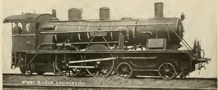
COMPOUND INSIDE CYLINDER 4-4-2 ENGINE.
