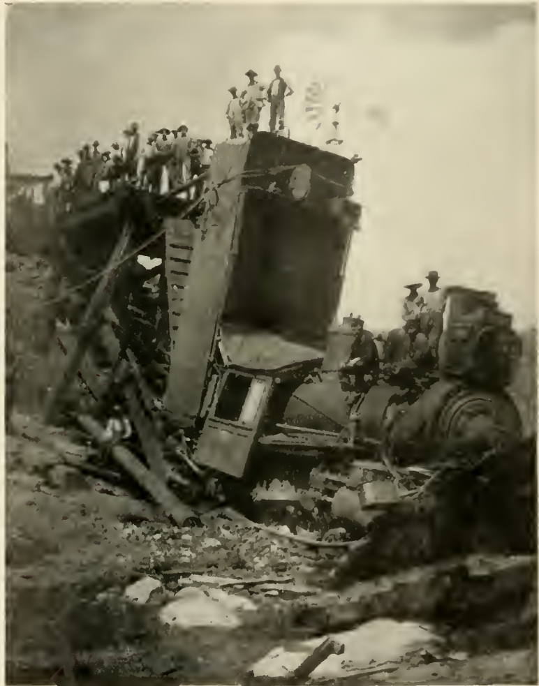
BRIDGE COLLAPSED WITH ENGINE TRYING TO START TRAIN
