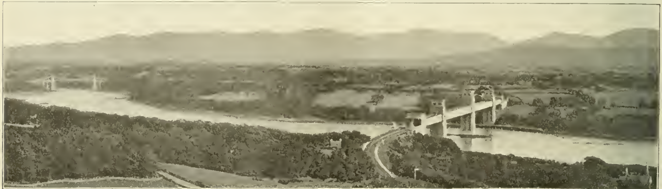
BRITANNIA TUBULAR BRIDGE OVER THE MENAI STRAIT.
