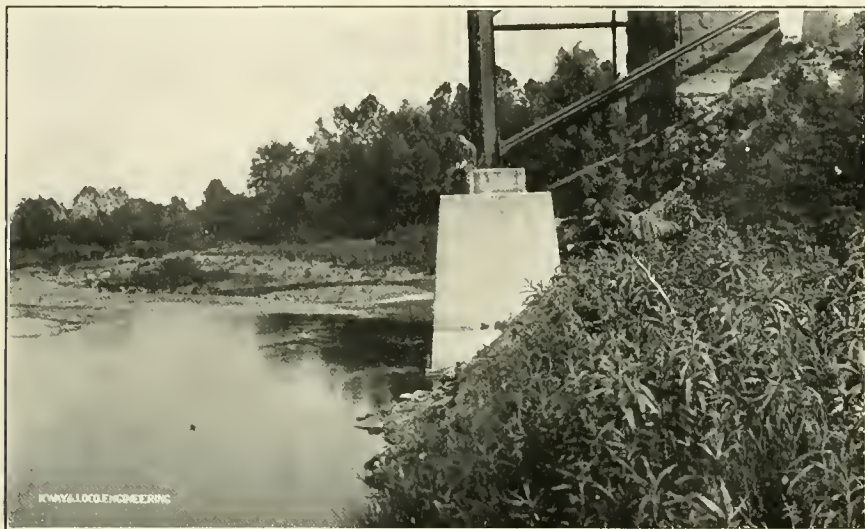
ABUTMENT OF GIRARD, PA., BRIDGE, NICKEL PLATE LINE.
