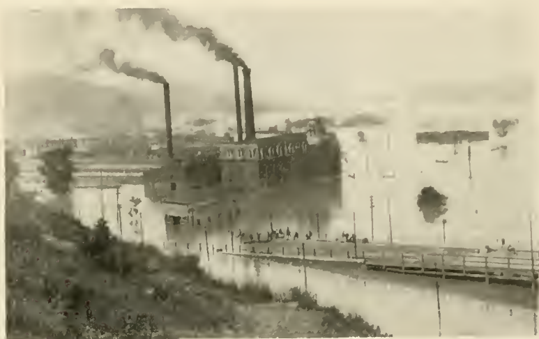
FIG. 5. THE KAW RIVER PUMPING STATION.
