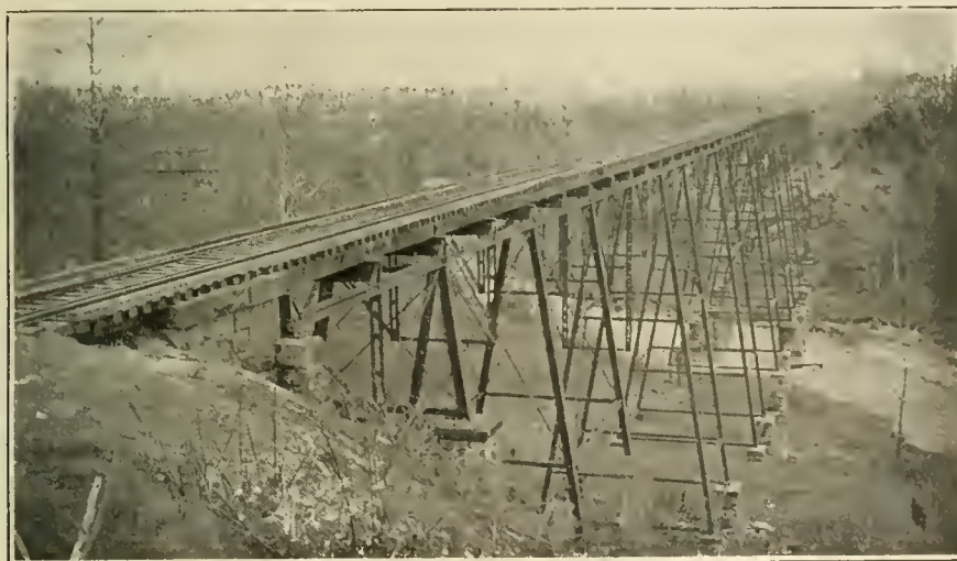
STATE LINE TRESTLE, NICKEL PLATE LINE.
