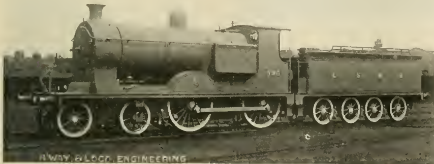
LONDON AND SOUTH COAST EXPRESS ENGINE WITH DRUMMOND BOILER.
