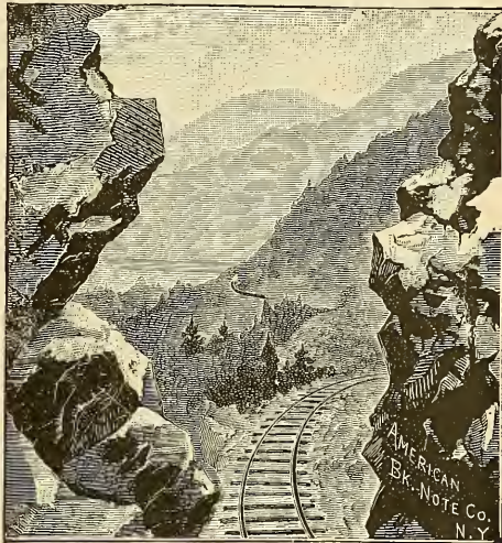
MAINE CENTRAL R.R.—THROUGH THE NOTCH.
