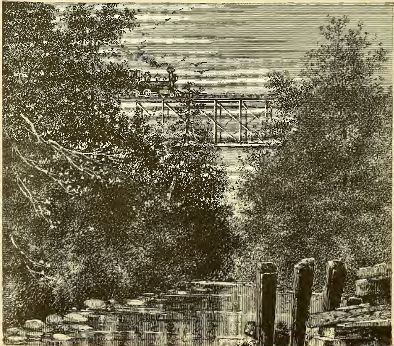
R., W. &amp; O. R.R.—MILL CREEK NEAR LOWVILLE.
