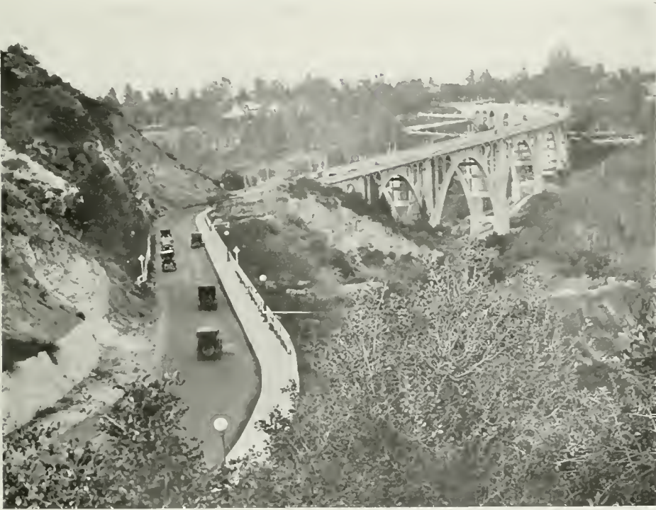
Linda Vista Bridge.
