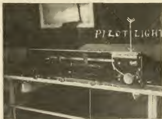
FIG. 1. Tubular pocket flash-light attached to Bucky-Potter Diaphragm.
