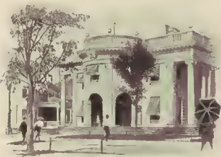
RHODE ISLAND BUILDING.
