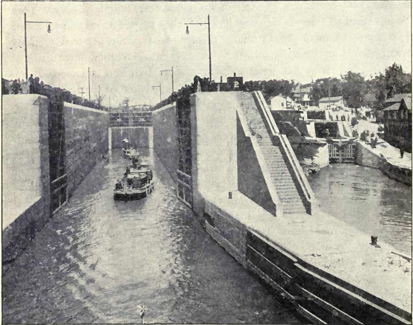
Above: First canal lock in New York State built at Little Falls (1796); length 70 ft., width 10 ft. Below: At right, three locks at Waterford after first enlargement of Erie Canal; length of each 110 ft., width of each 19 ft. At left, new Barge Canal lock replacing three locks at right, length 328 ft., width 45 ft.
