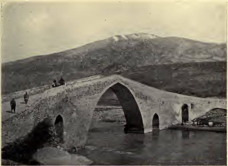
Old Bridge over the Jihon on road to Zeitún.
