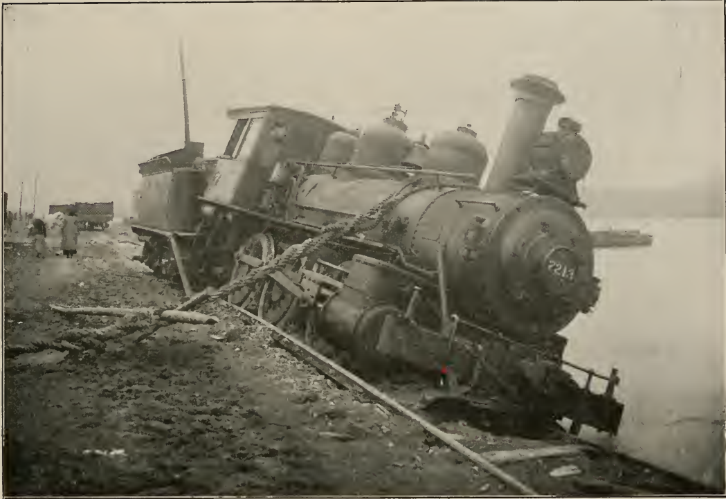
CAVING OF THE LEVEE AT LAWRENCEBURG, INDIANA—BIG FOUR ENGINE IN DANGER
