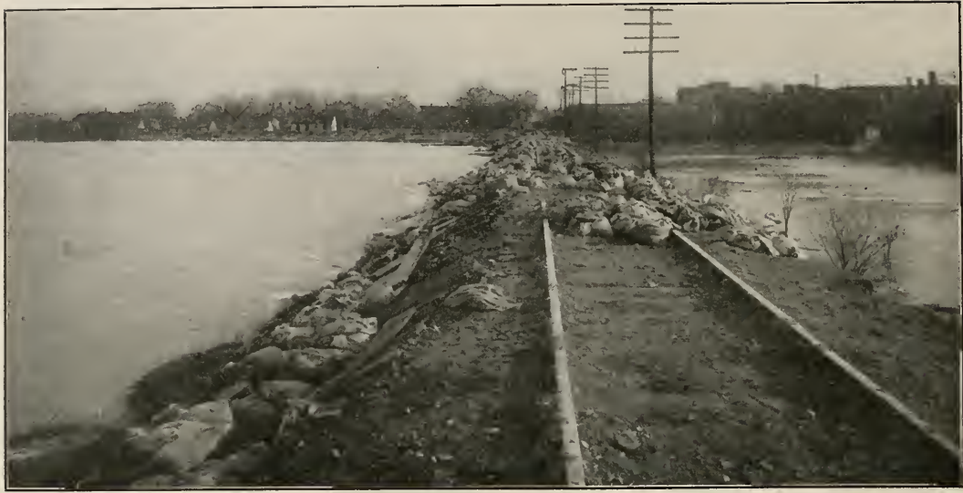
THE LEVEE AT LAWRENCEBURG, INDIANA, BEING STRENGTHENED WITH BAGS OF SAND
