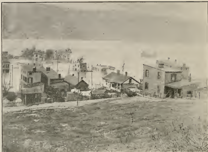
OHIO RIVER OVERFLOW, CINCINNATI, OHIO
