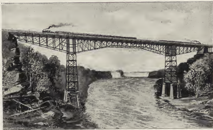
CANTILEVER BRIDGE OVER NIAGARA RIVER
