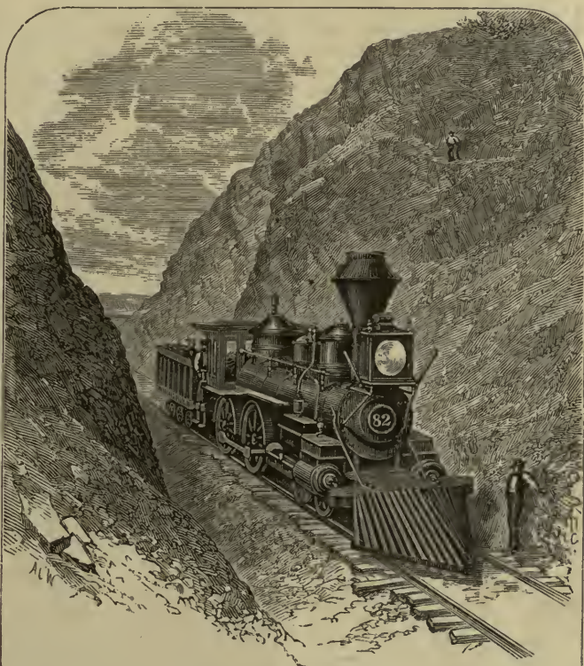
ROCK CUT, NEAR ASPEN.
