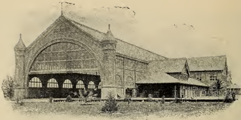
ARCADE DEPOT—LOS ANGELES.
