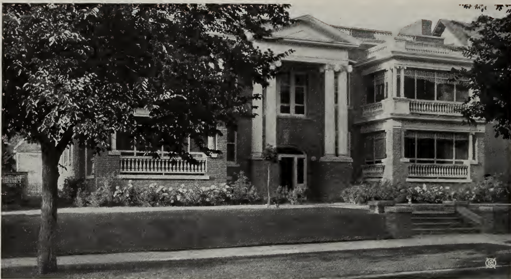
The planting of Shrubs around the foundation of a flat building makes it more homelike
