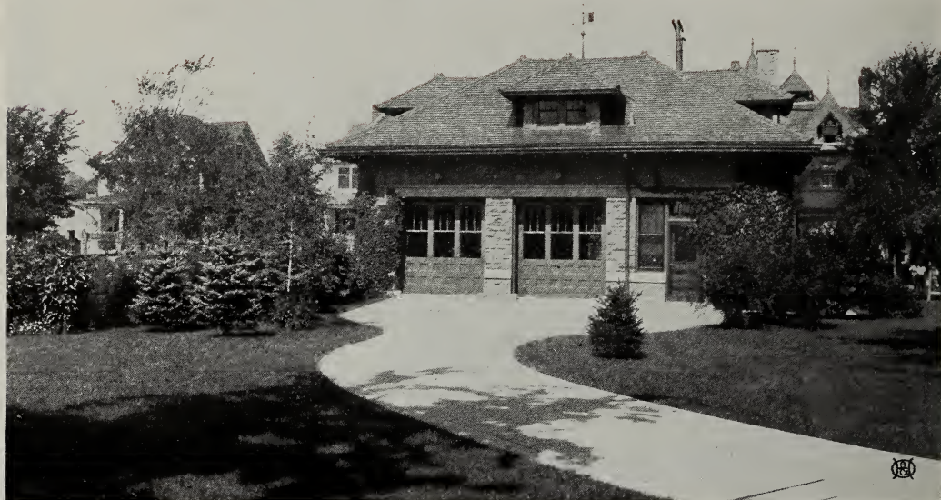
The Spruces, Shrubs and Vines are arranged to add to the architectural design of the garage
